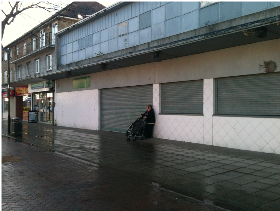
Existing internal front shutters – Park Parade, Leigh Park
