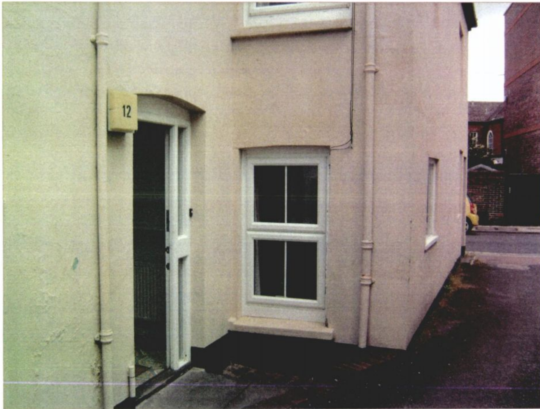
Side elevation with access door
