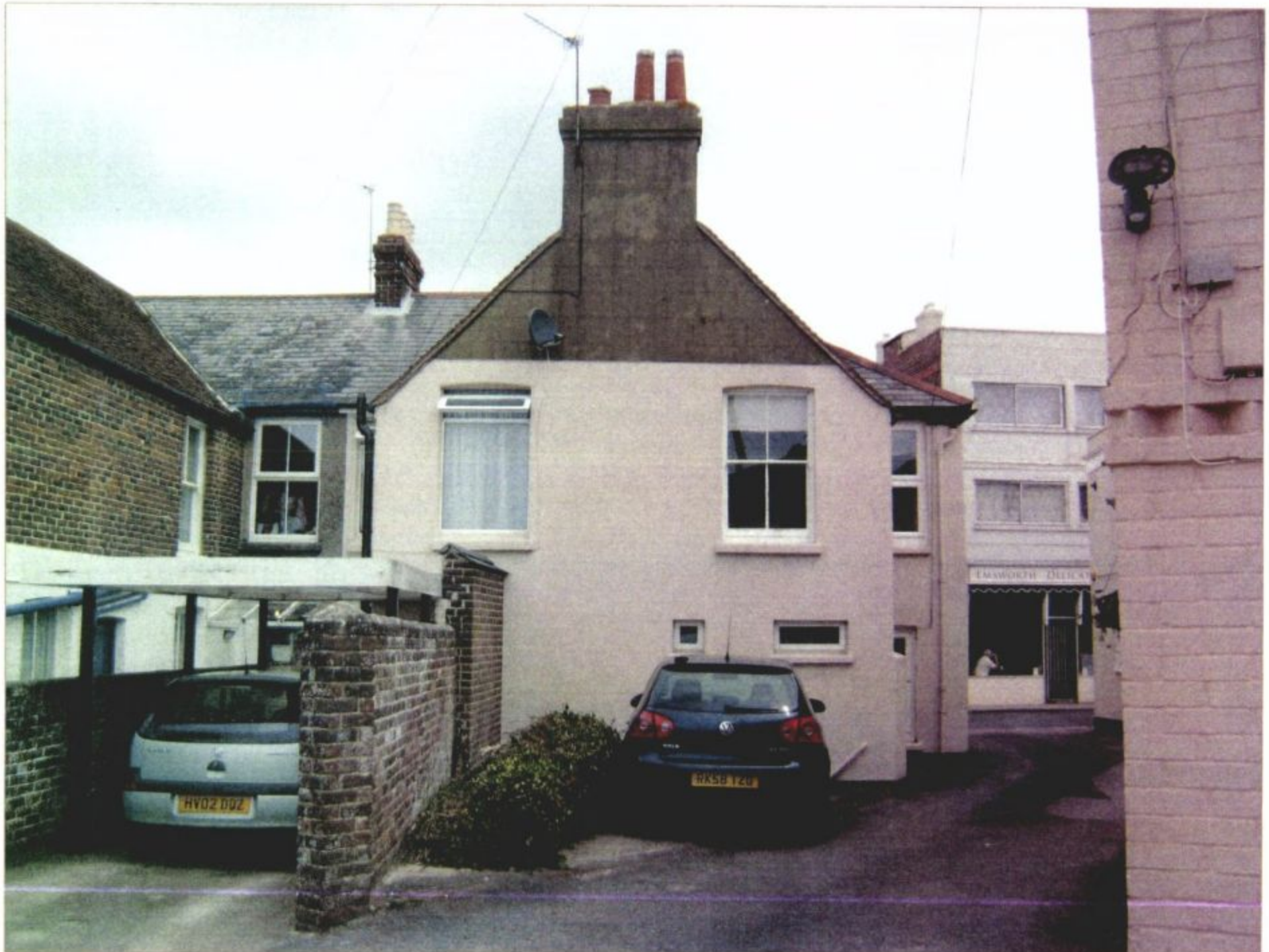
Rear elevation showing car parking space
