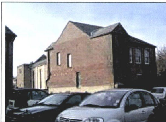
Current view of rear elevation-1
