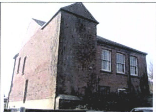
Current view of rear elevation-2
