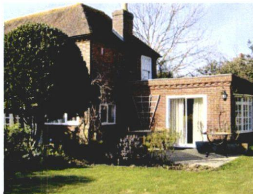
Rear Elevations Eastney House
