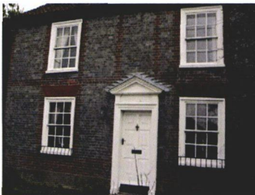
Front Elevation Eastney House
