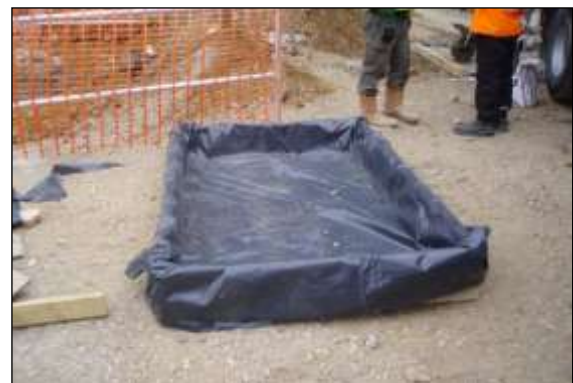
Photo 47: Soil bunding or a supporting framework covered in heavy-duty plastic sheeting is essential where there is a risk of spillages contaminating RPAs. This specifically applies to
