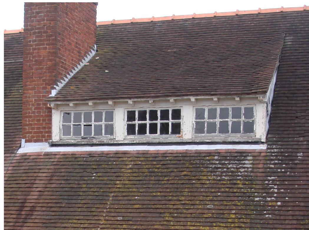
RECENT PHOTOGRAPH OF THE SOUTH WEST ELEVATION SHOWING THE EXISTING MULTI WINDOW DORMER WITH A PITCHED PLAIN TILE ROOF
