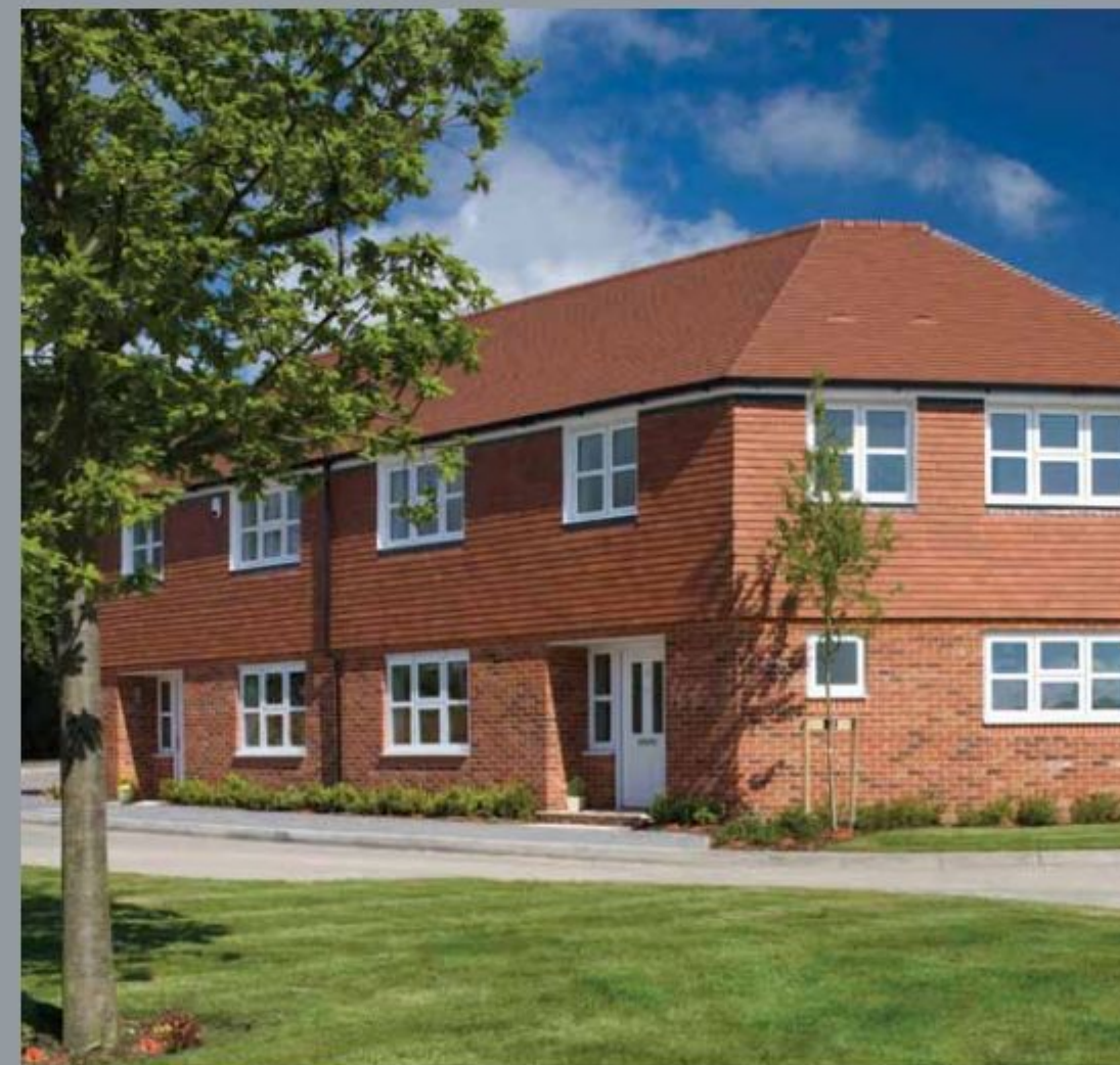
Existing Linden Homes development
