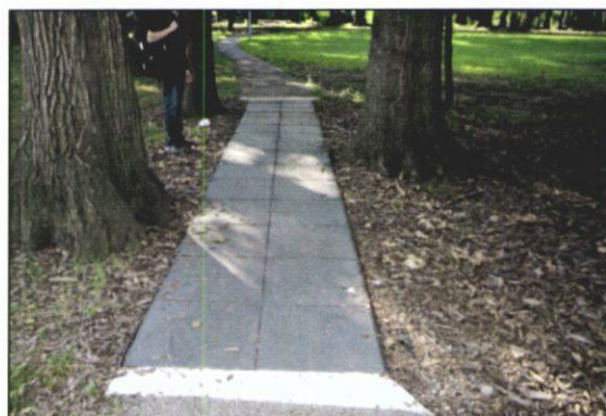
Photo 33: Where surfacing is needed close to rapidly growing buttress roots, a light metal frame with rubberised surfacing will allow the path to distort without cracking as the roots grow.
