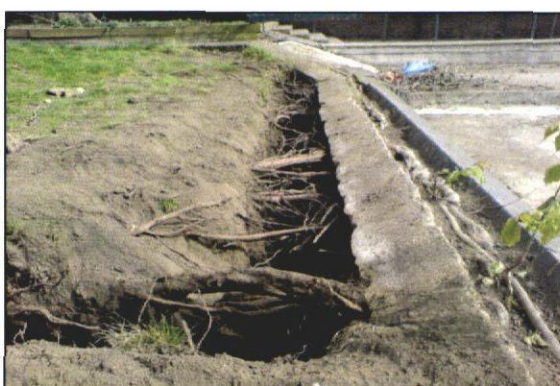
Photo 17: Air spades are particularly useful where roots are very dense.
