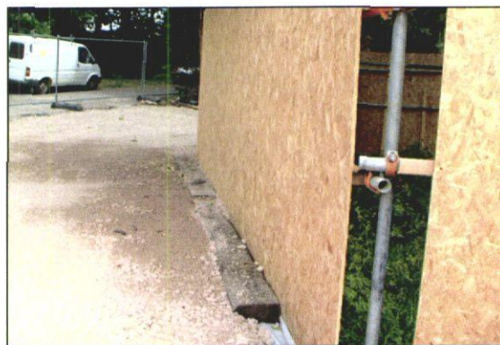
Photo 27: Although this is only a temporary surface, railway sleepers pinned into the ground can be used to retain the edges of new surfacing.
