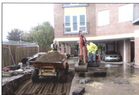
Photo 53: Structural tree soil retains sufficient structure for tree roots to grow, even when compacted.
