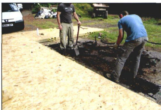
Photo 15: Careful hand-digging using conventional tools is acceptable for exposing roots in RPAs.
