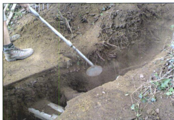
Photo 16: Air spades are very effective at exposing roots and services with minimal damage.
