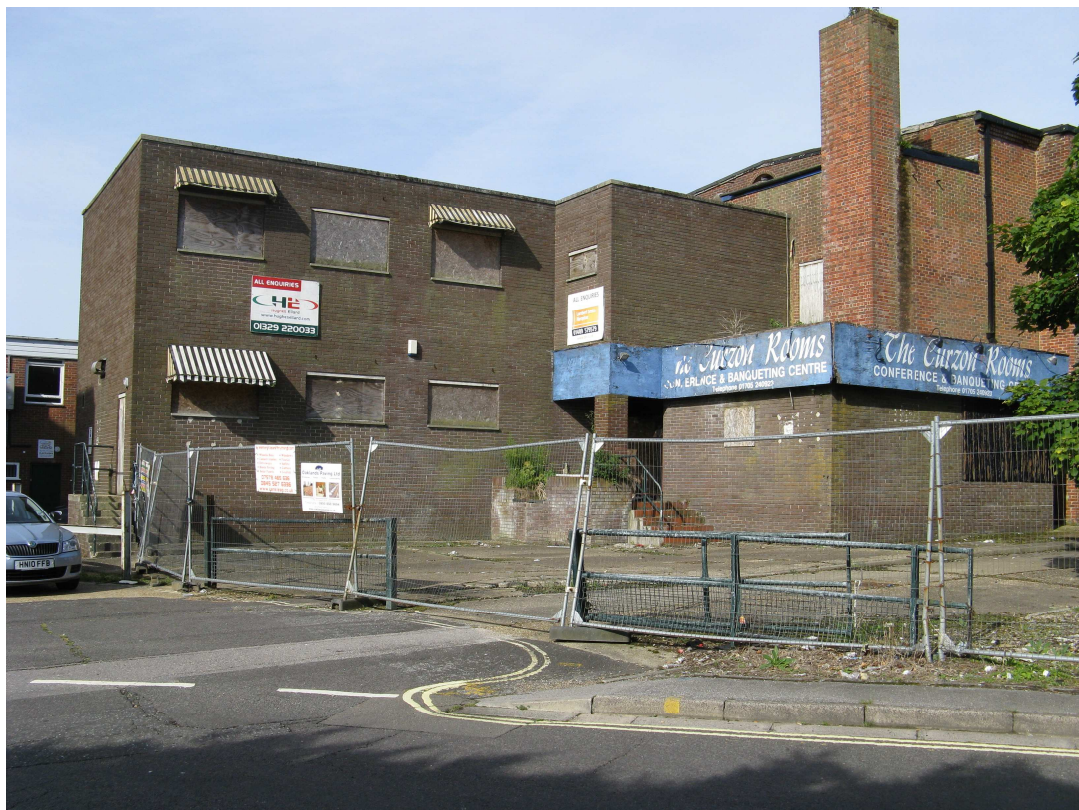
Photo 3 Agglomeration of buildings at the rear facing Curzon Road
