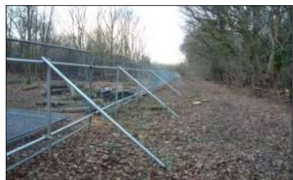
Photo 2: Heras fencing wired to scaffold braced posts is a robust and effective interpretation of the BS specification.
