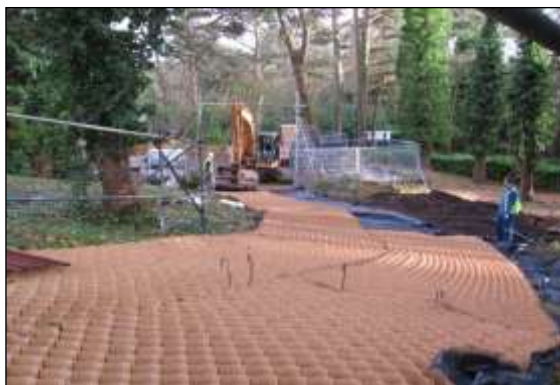
Photo 24: The three-dimensional cells are opened up, spread across the area to be surfaced and pinned in place ready for the stone filling.
