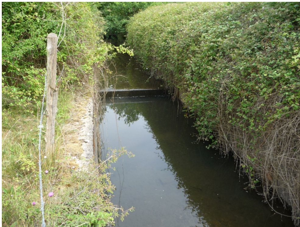
Photograph 1 - Northern canalised section of the Hermitage Stream showing concrete sides of culvert with overhanging bramble
