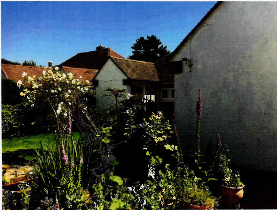
Existing House – Extension is proposed where the gable is to the right hand side of this photo.
