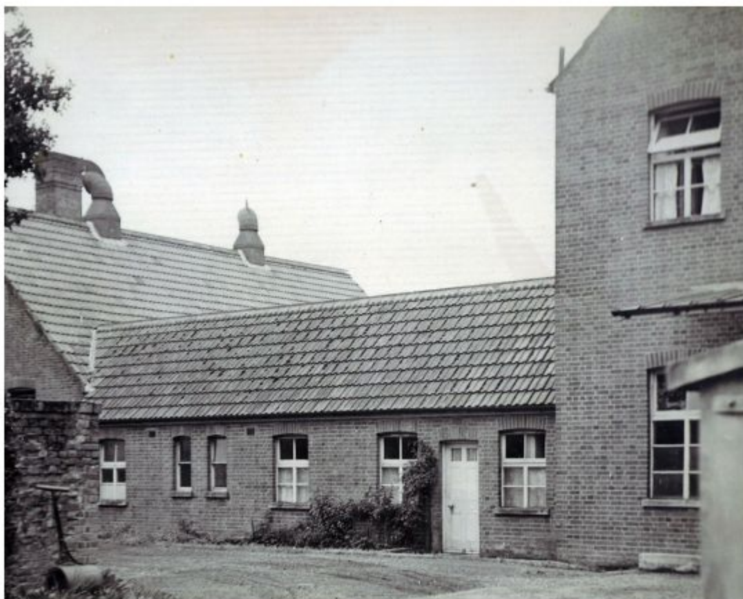
Convent link to Laundry Block.
