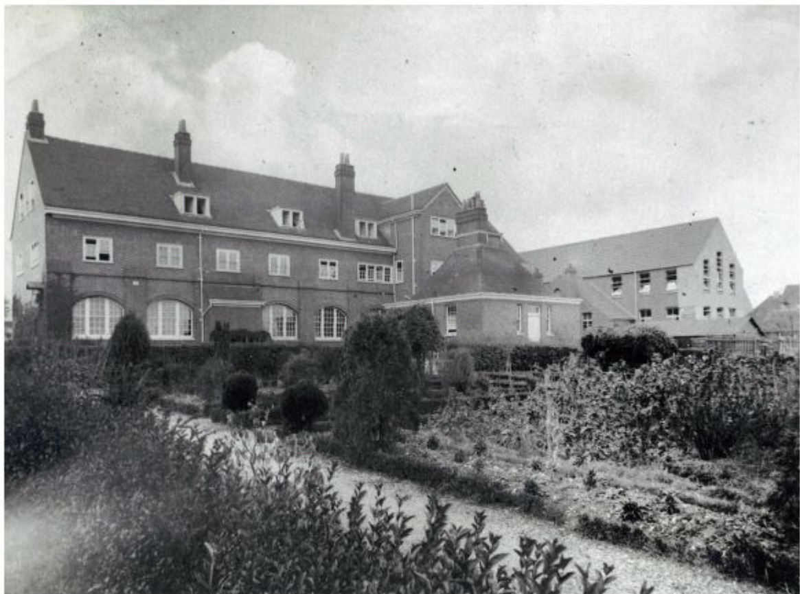
East elevation of Convent.
