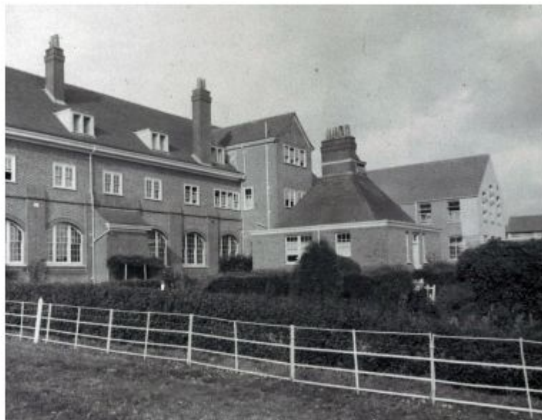
Figure 3.7. View of rear of Convent across gardens.
