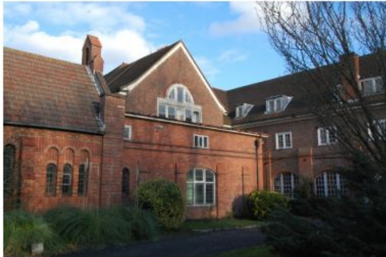
Figure 4.4. Corridor connecting Chapel and Convent.
