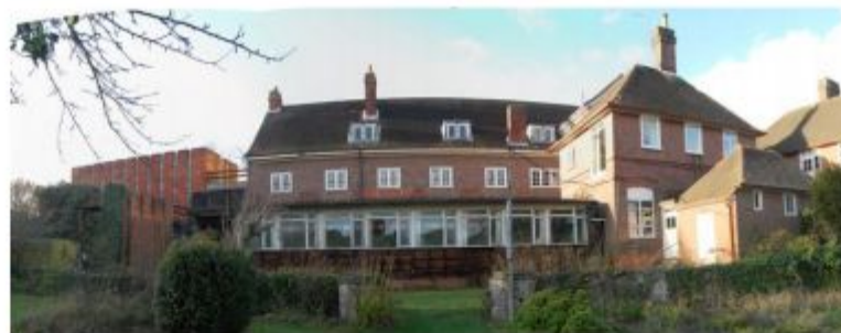
Figure 4.2. Single storey structure to rear.
