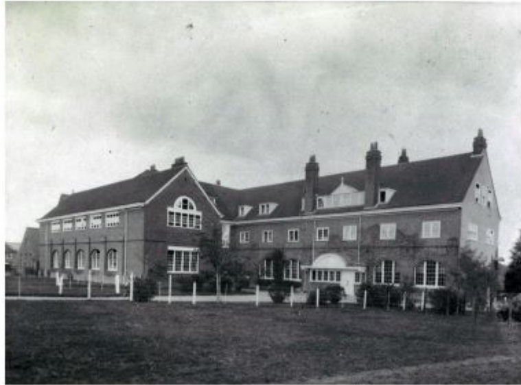
Figure 3.1. West elevation of convent.
