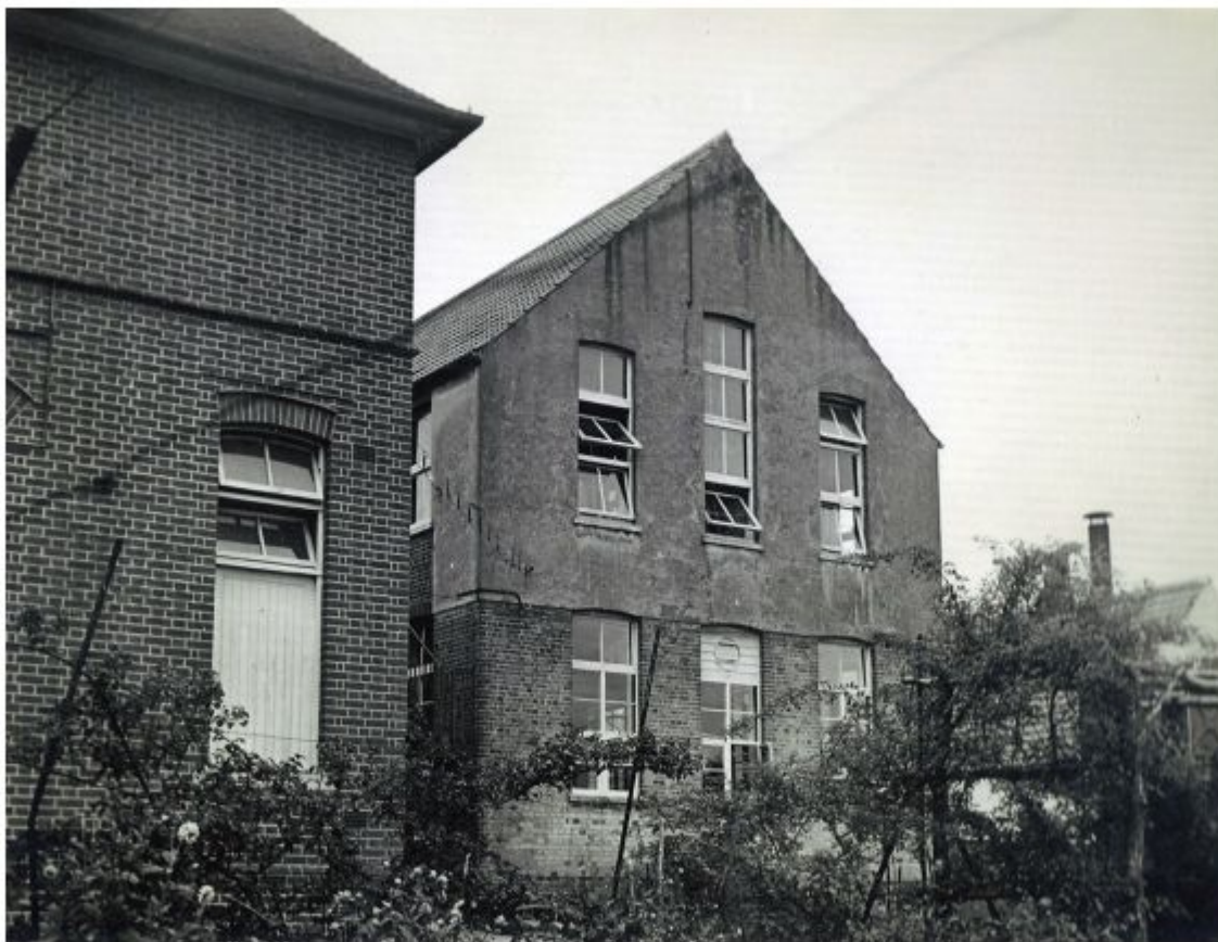
East elevation of dormitory.
