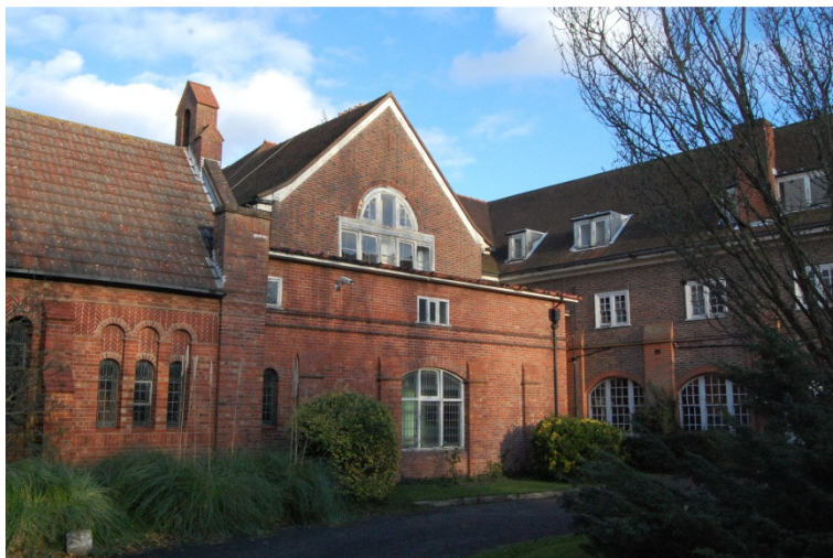
Figure 4.4. Corridor connecting Chapel and Convent.
