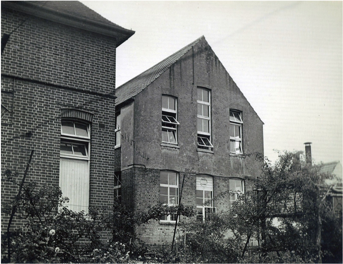
East elevation of dormitory.
