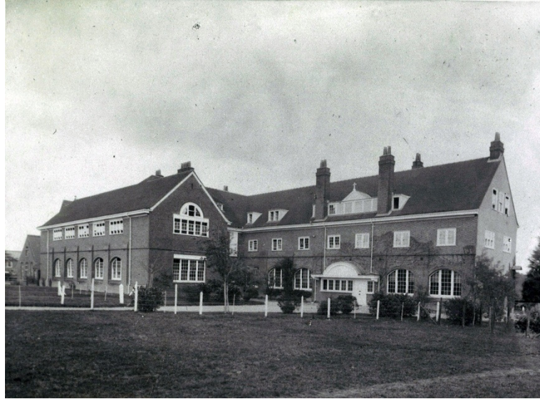
Figure 3.1. West elevation of convent.
