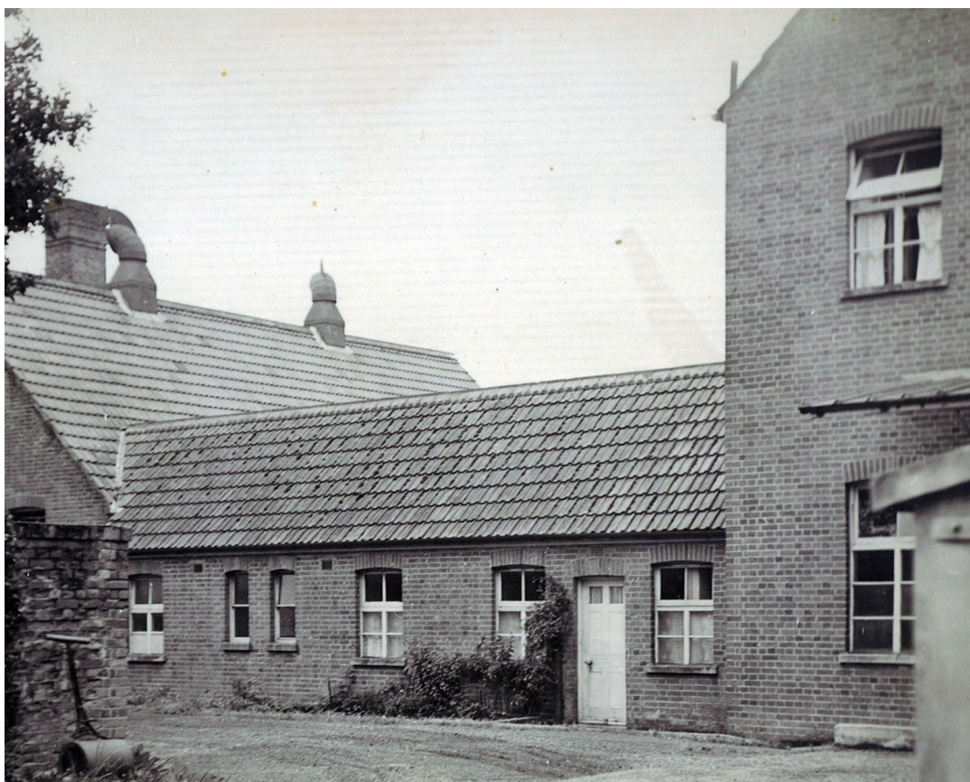
Convent link to Laundry Block.
