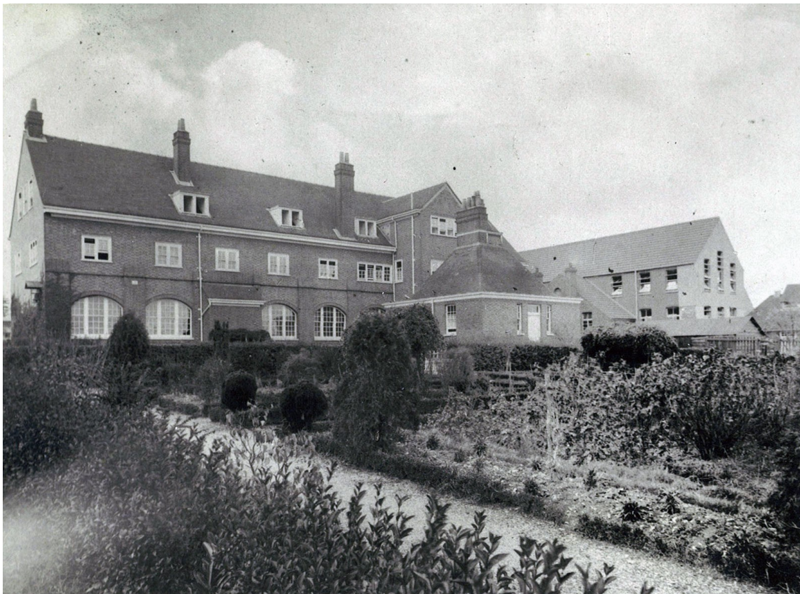
East elevation of Convent.
