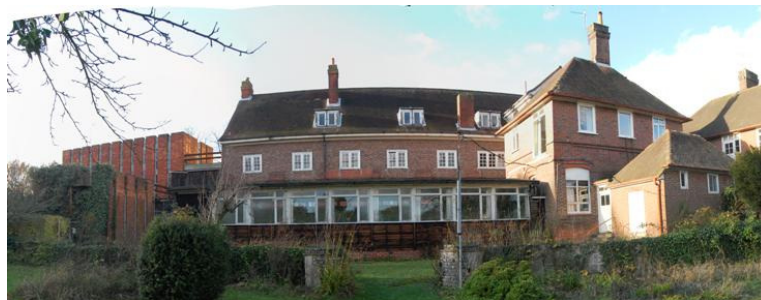
Figure 4.2. Single storey structure to rear.
