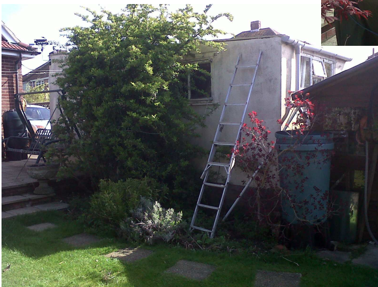
Above and left, existing garage and it's location at the rear of No. 1 Springfield Close.
