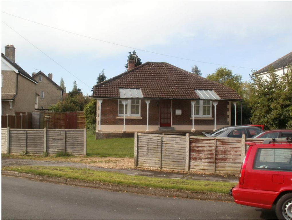
Application Photographs Redevelopment of 20 The Crescent Purbrook. Front elevation 20 The Crescent
