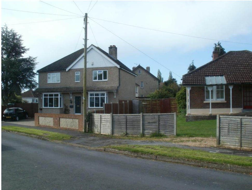
Front elevation of no 22 The Crescent
