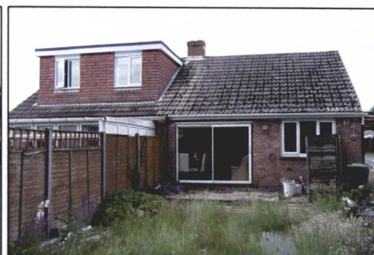
Existing South West Elevation Image
