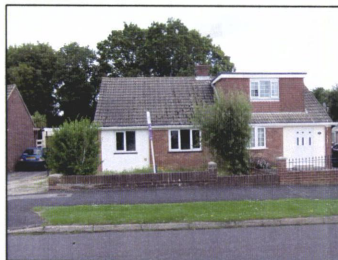
Existing North East Elevation Image
