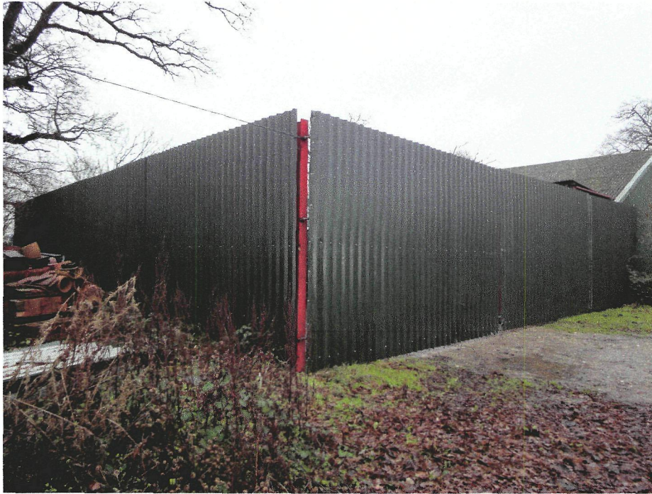
View from South west facing North east showing new fence in relation to existing shed
