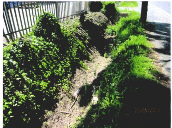
General poor state of watercourse
