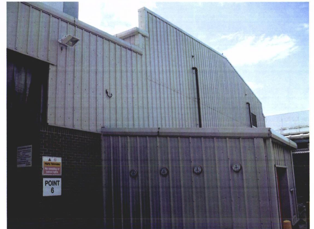
View of West (1) Elevation
