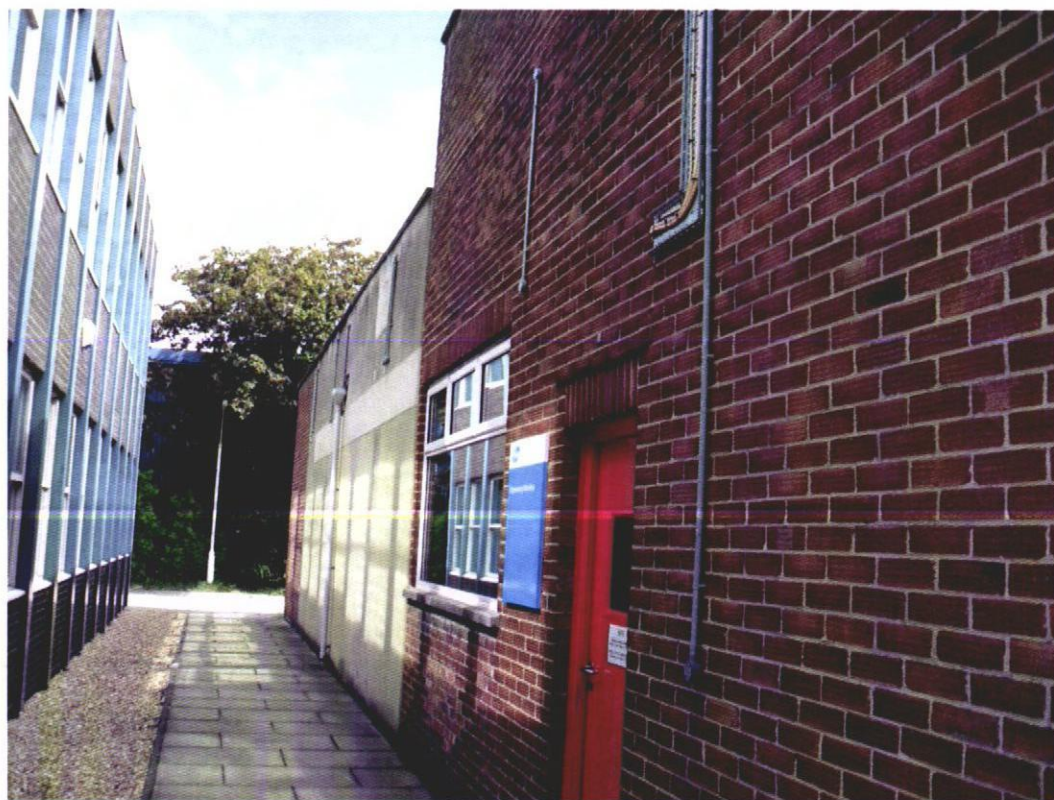
View of West Elevation
