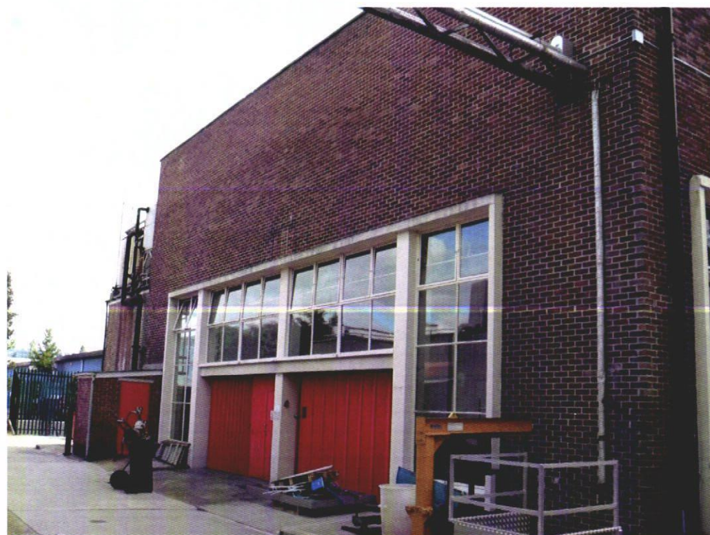
View of West Elevation
