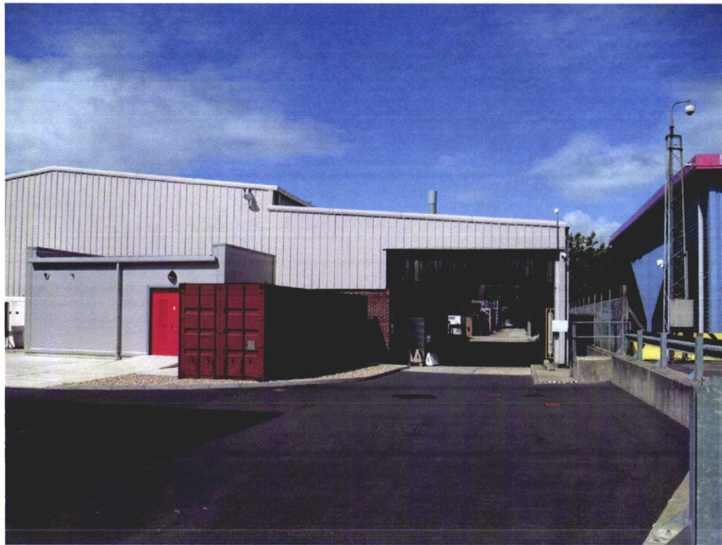
View of East (1) Elevation
