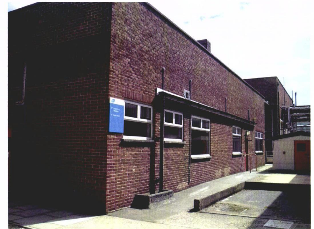
View of South Elevation
