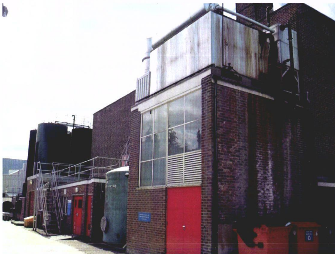
View of North Elevation
