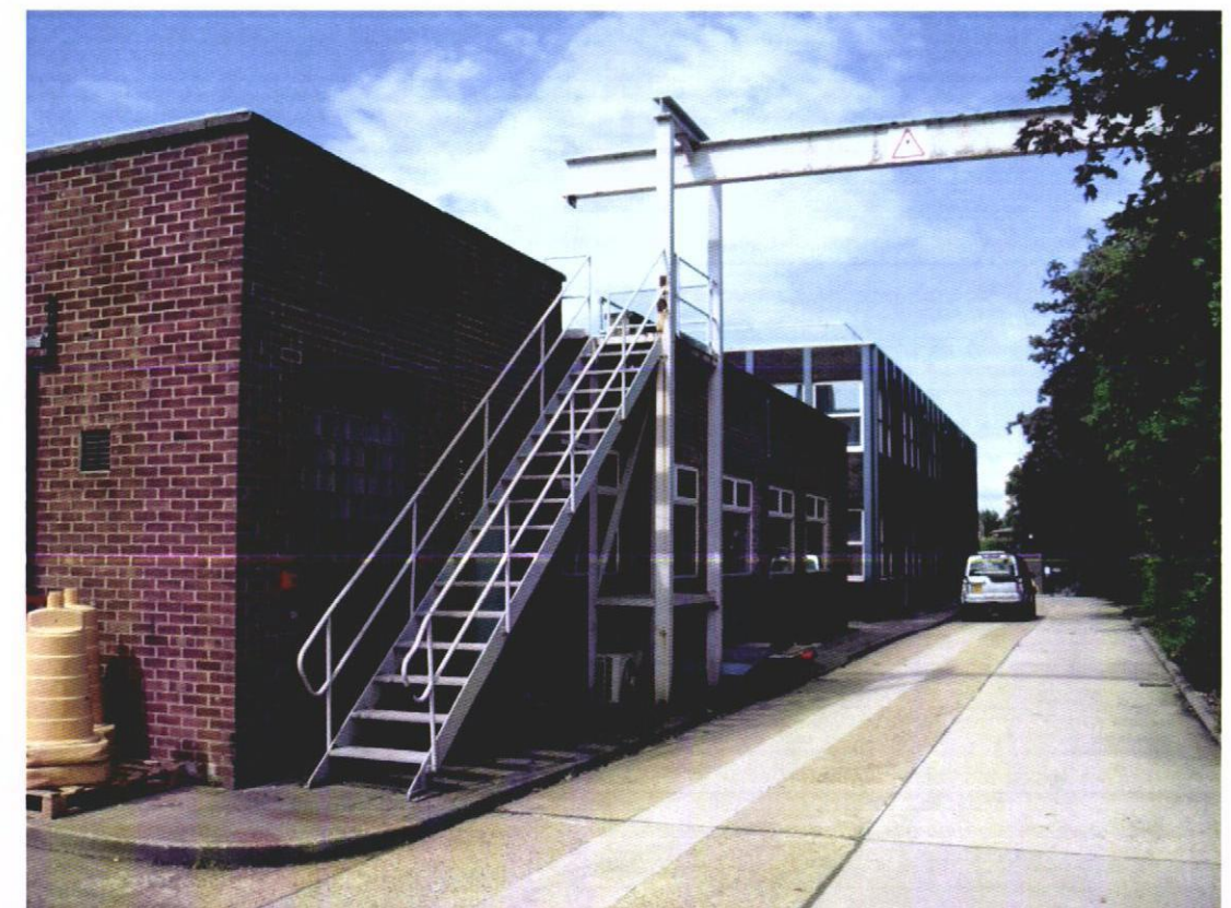
View of North Elevation
