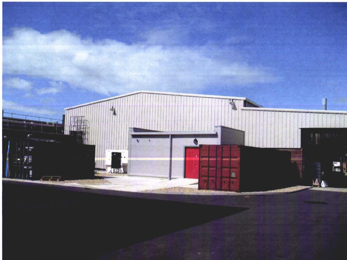
View of East (2) Elevation
