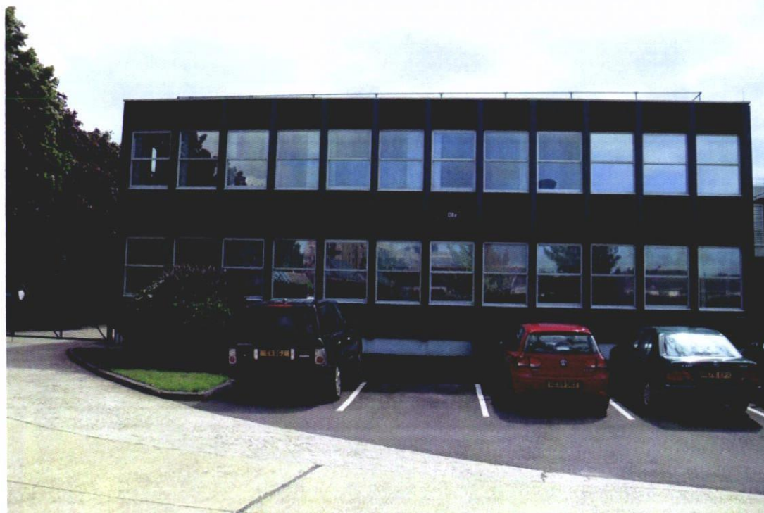
View of West Elevation
