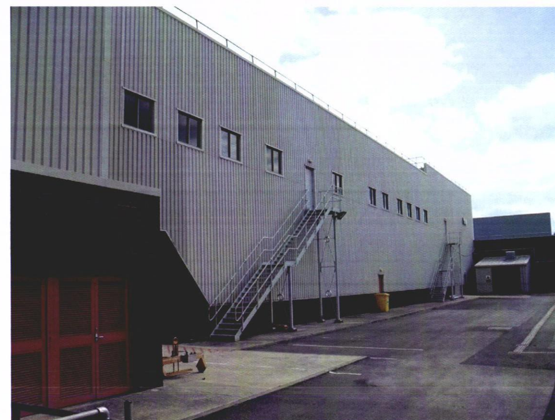
View of South (1) Elevation
