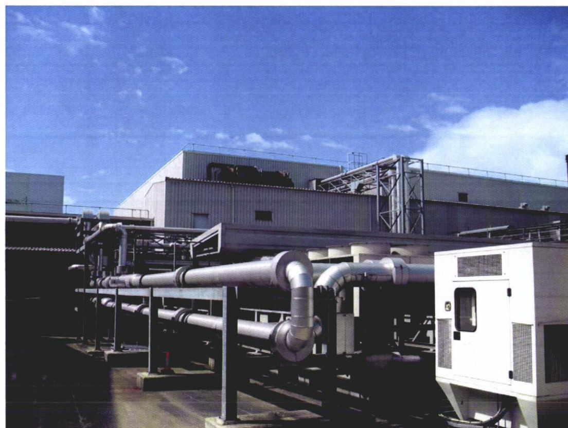
View of North Elevation
