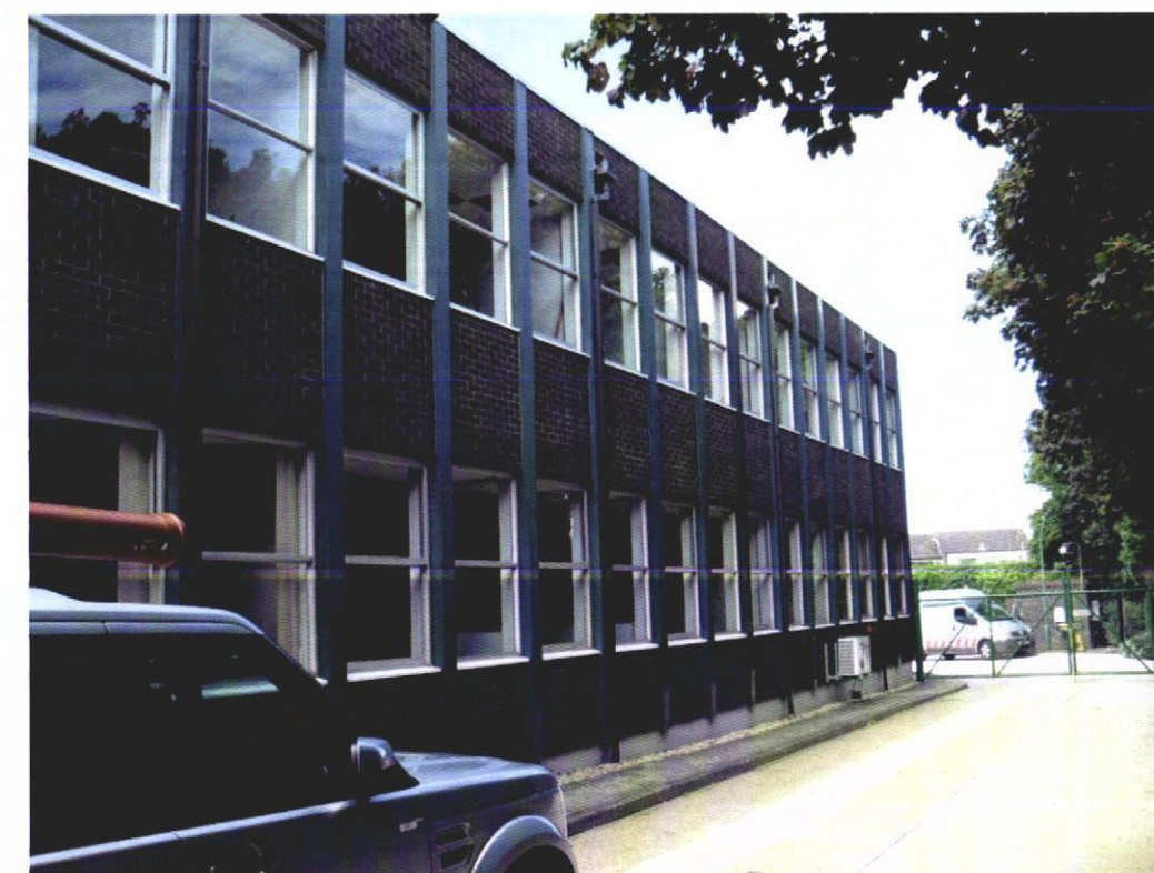
View of North Elevation
