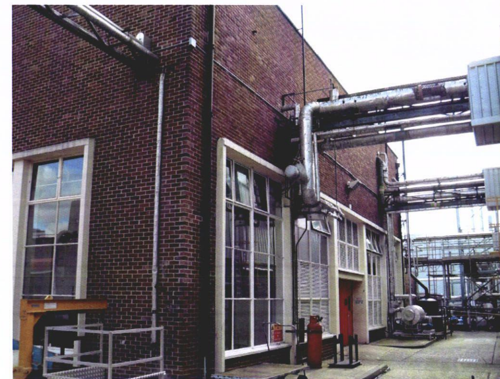
View of South Elevation
