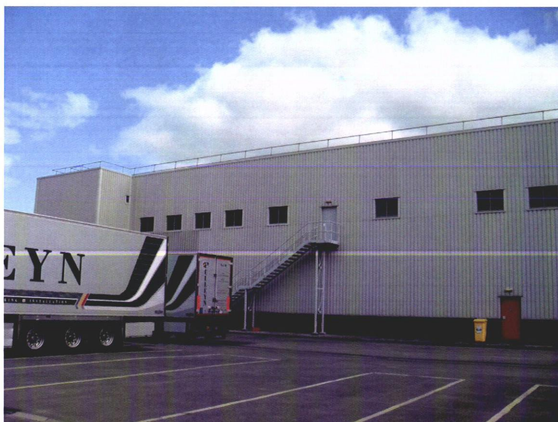
View of South (2) Elevation
