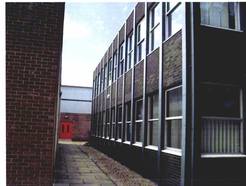
View of East Elevation
