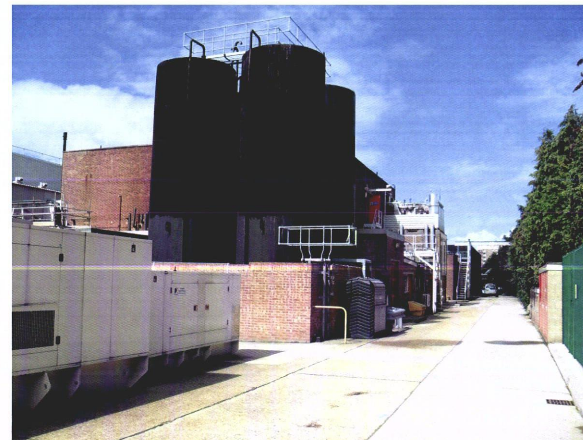
View of East Elevation
