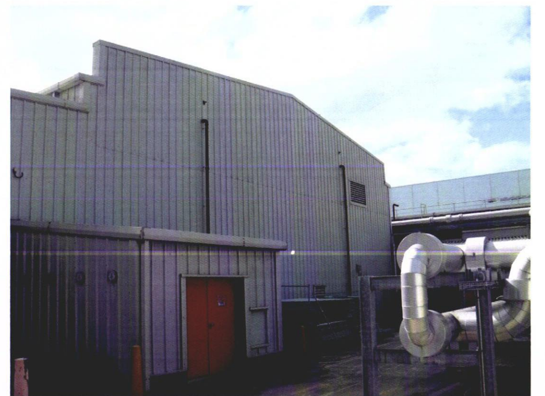
View of West (2) Elevation
