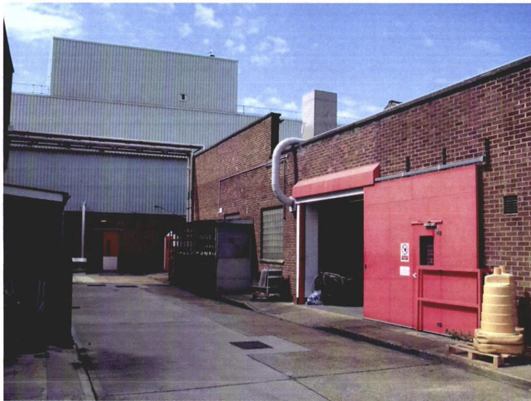
View of East Elevation
