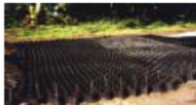
Expanding and staking Geoweb panels
