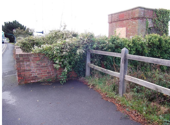
Approach side of building and wall where wall will be removed.
