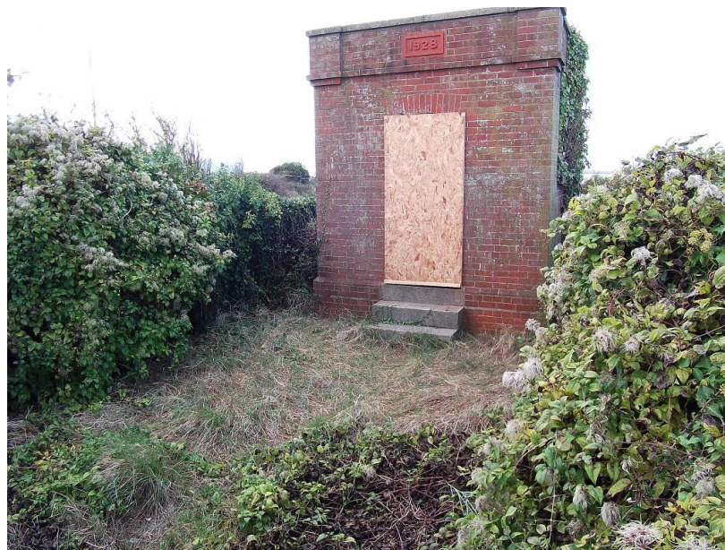
Front view of Brick building to remain
