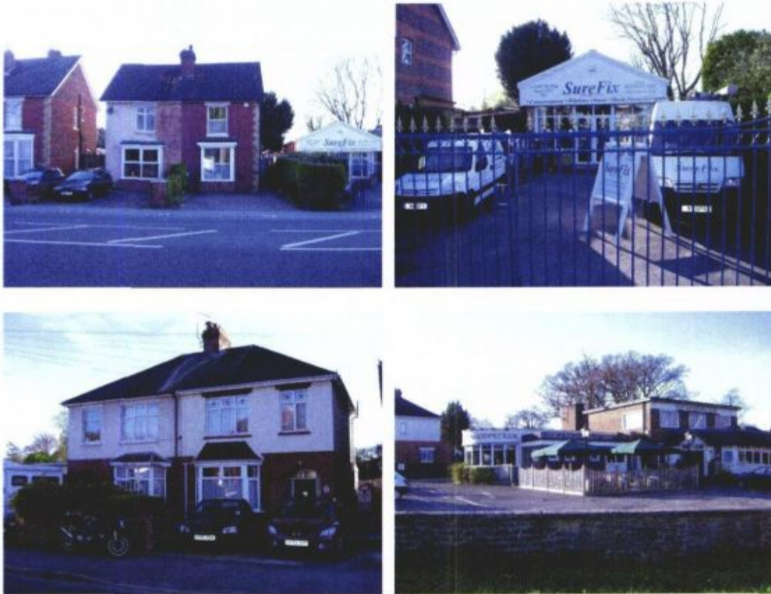
Fig 4. Existing site photos
