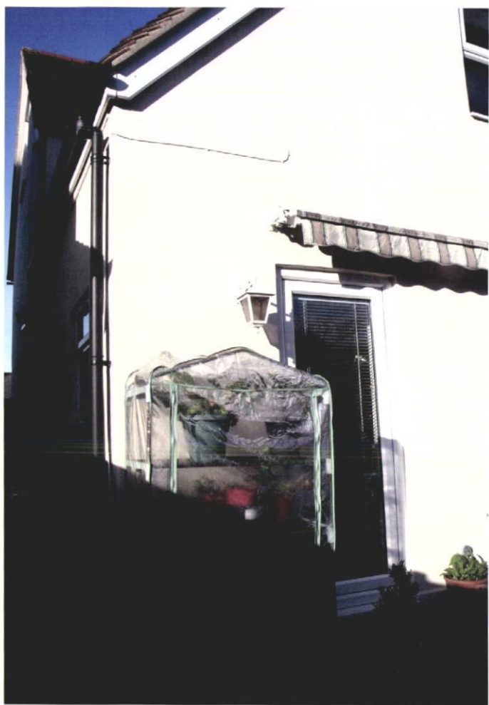
6 STANLEY ROAD CORNER REAR & SIDE
