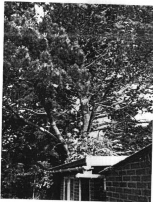
Figure 6 –Pine tree, looking south-east. Note lack of growth/vigour in middle of tree.
