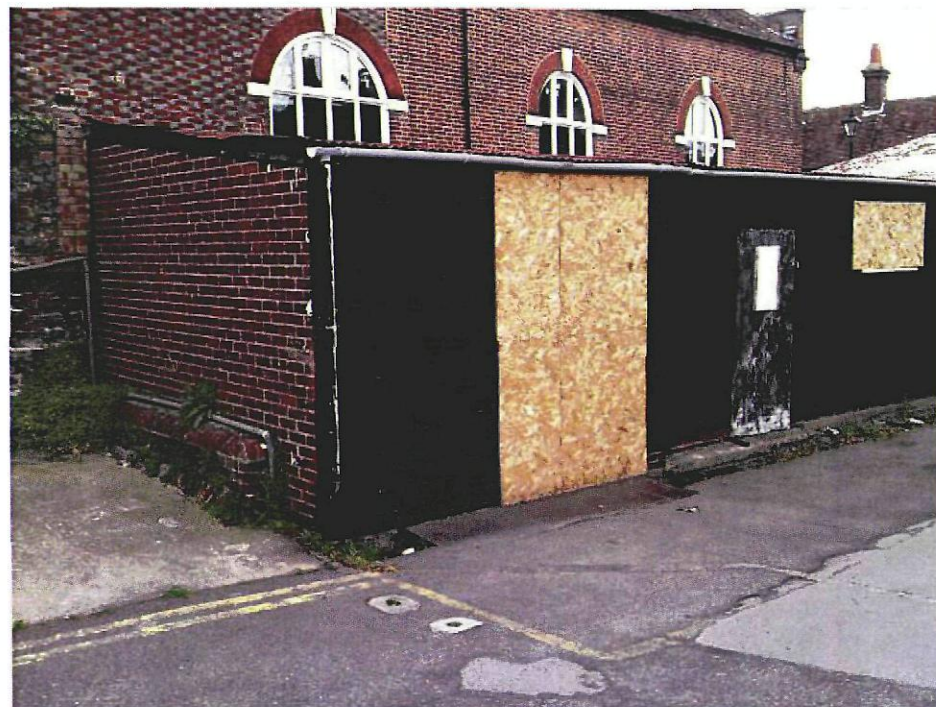
Existing East Elevation, timber outhouse building
