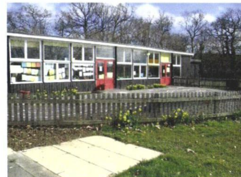
4 West elevation (rear) of southern classroom wing (adjacent Hooks Row)
