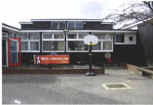
1 Central section of east elevation (facing Barncroft Way)
