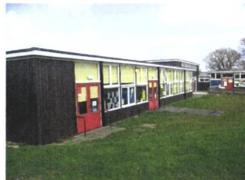
5 South elevation (rear) of western classroom wing
