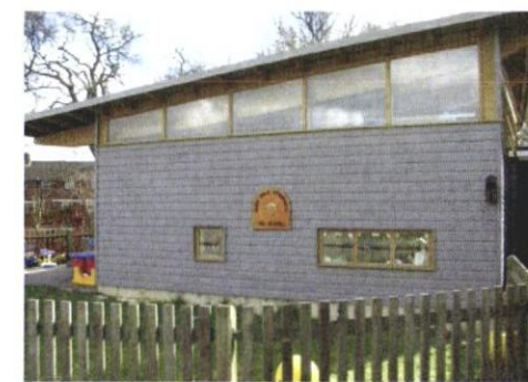
9 North elevation of pre-school
