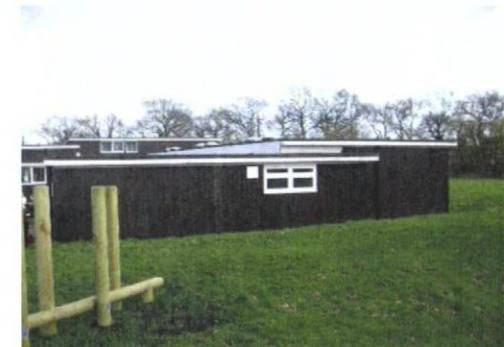
3 Western (end) elevation of western classroom wing
