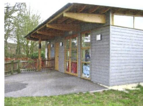
8 East elevation of pre-school
