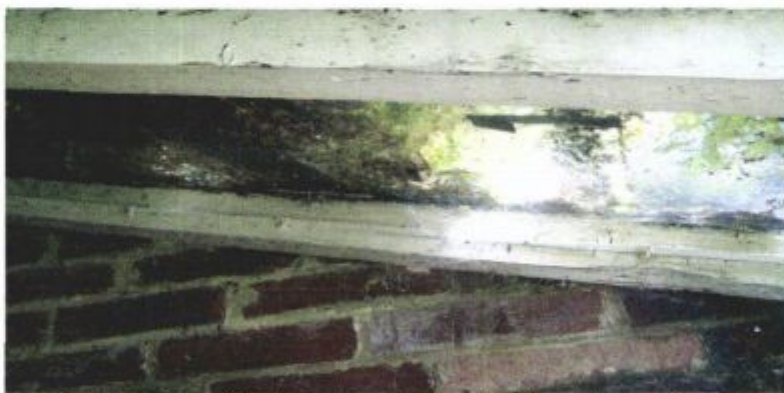
Interior of glazing and rafter against boundary wall
