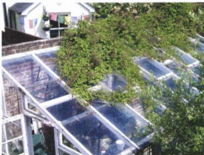
View of existing roof and north boundary wall
