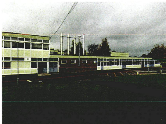
Fig. 4 Typical SCOLA elevations. Area between main campus and the sports/drama block.
