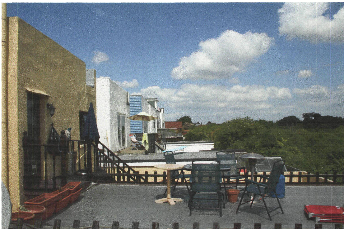
23 Sandy Beach (foreground) showing 1 st floor level outside area and balcony and stairs. Beyond this is 22 Sandy Beach Estate showing Balcony and used roof area. Beyond this is 21 with a balcony. Beyond this is a further large wooden balcony see further photograph.
