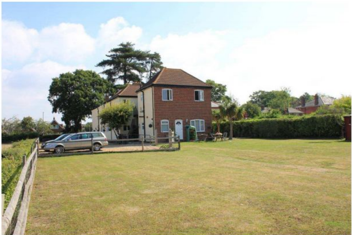
Photo 4 – View looking east towards the existing south-west elevation of the hotel.
