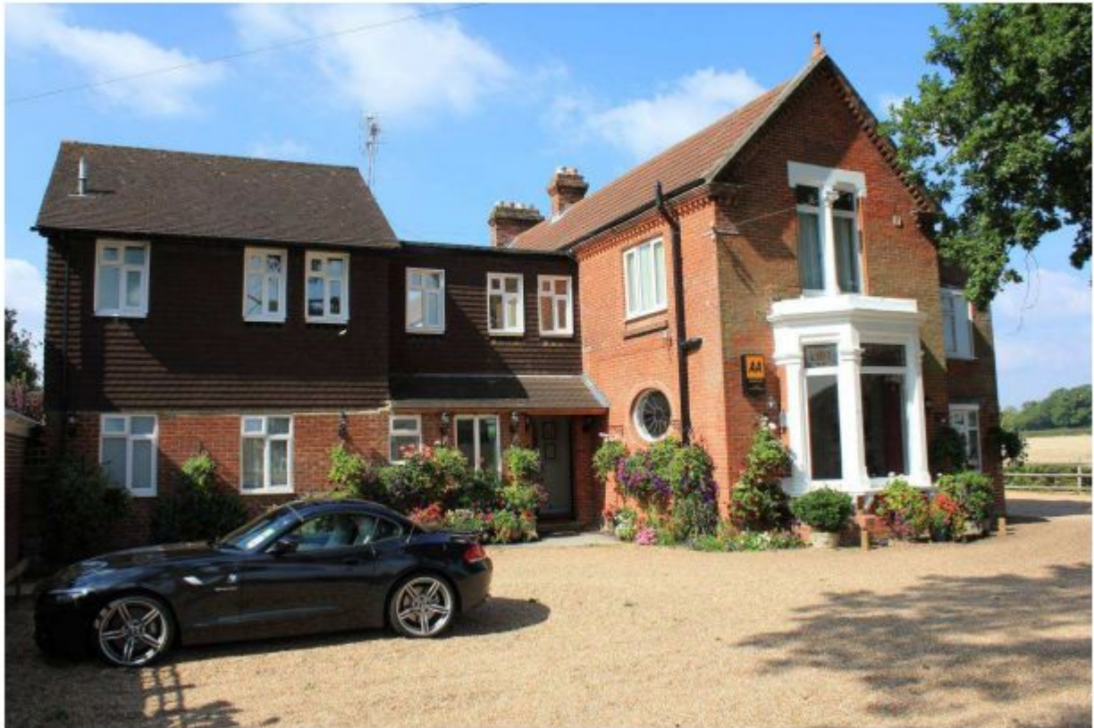
Photo 1 –Main entrance to hotel and north-east elevation..
