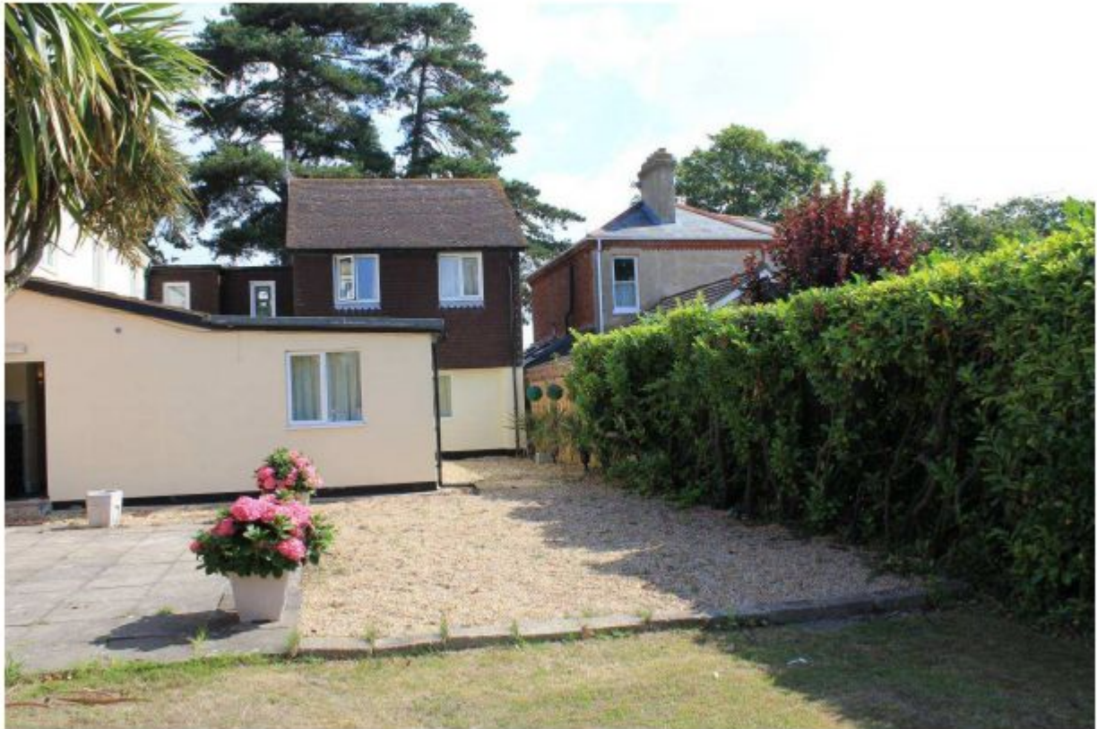
Photo 7 – View looking east at the rear of the hotel showing No. 75 right of centre, adjoining the site.
