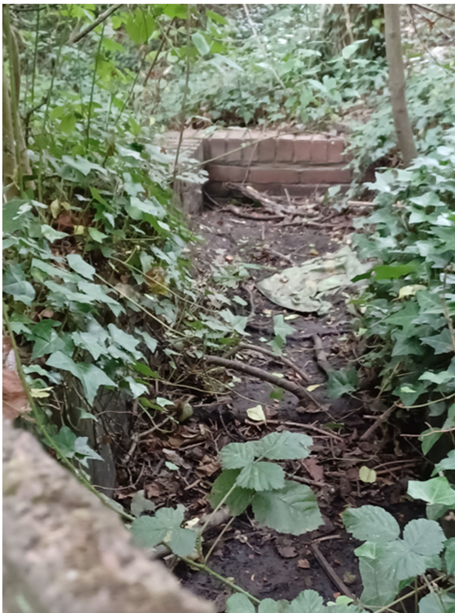
Figure 5.2: Approach to culvert
