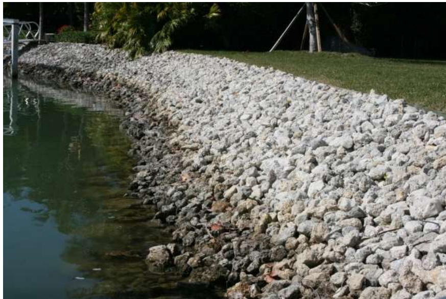
Figure 5. - Example of riprap on a riverbank [1]
