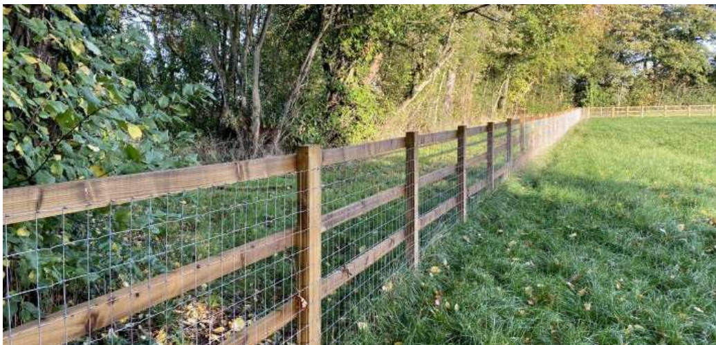
Figure 6. - Typical livestock proof post and rail fence [2]
