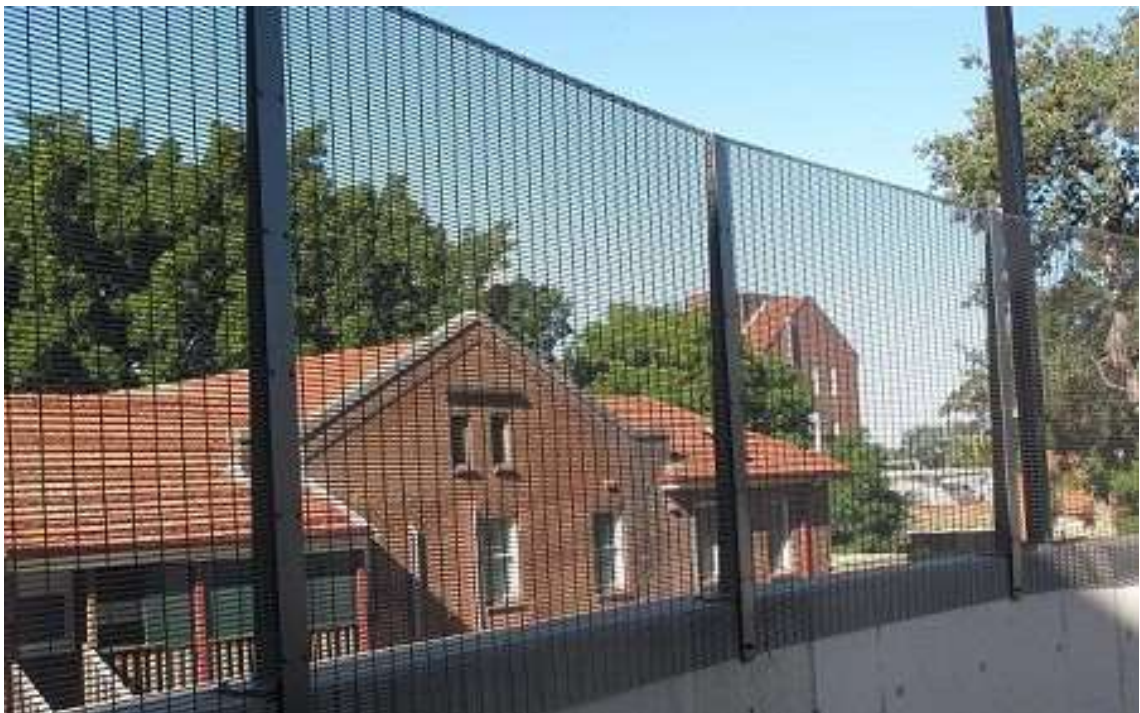
Figures 9a & 9b. - Example anti-climb fencing [3]
