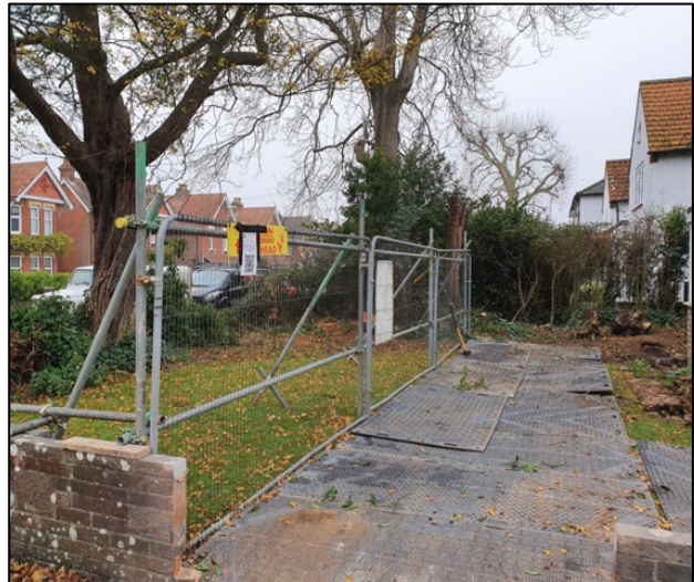
GP2: Tree protection barriers & trackmat ground protection
