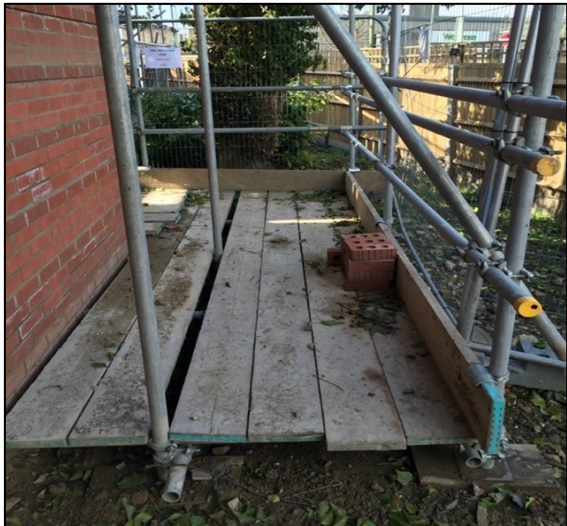
GP1: Tree protection barriers and scaffold ground protection
