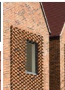
Projecting Brickwork Feature
