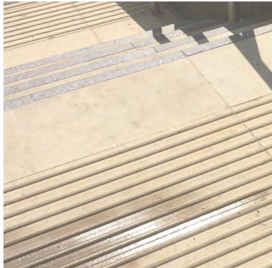
Accessibility - suitable tactile corduroy paving
