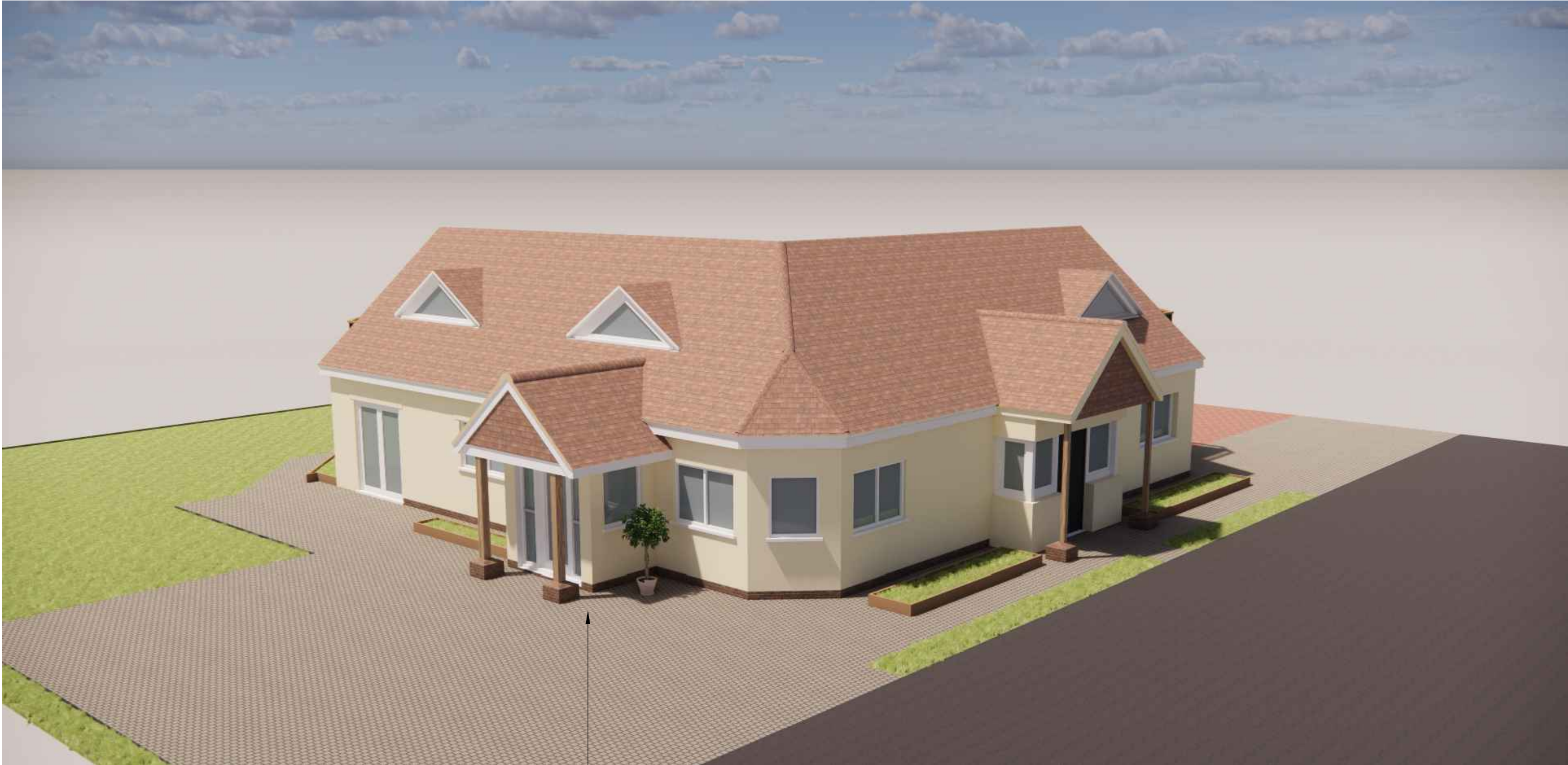
New Porch Extension
