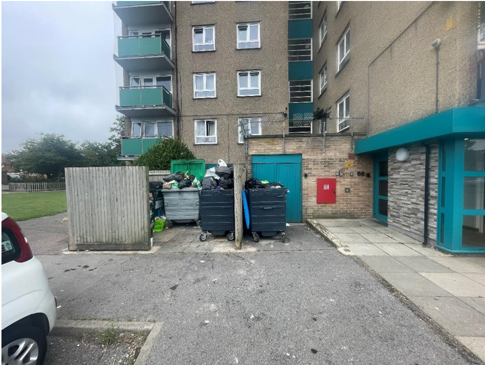
Photo 01 Showing current refuse store location (Solent House East Elevation)
