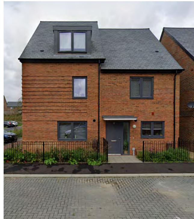
Projecting brick detailing, red brick facade, dark window and doors.
