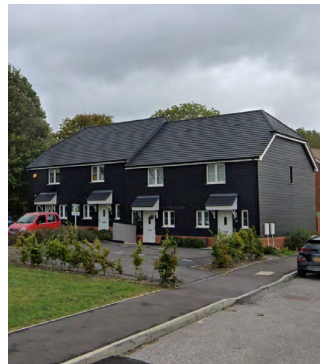
Brick plinth with dark weatherboarding, door canopy, white windows.
