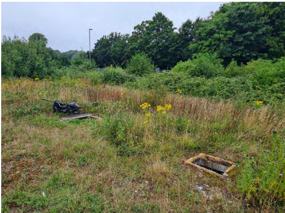
Plate 7: Two open manhole covers were located along the western edge of site.
