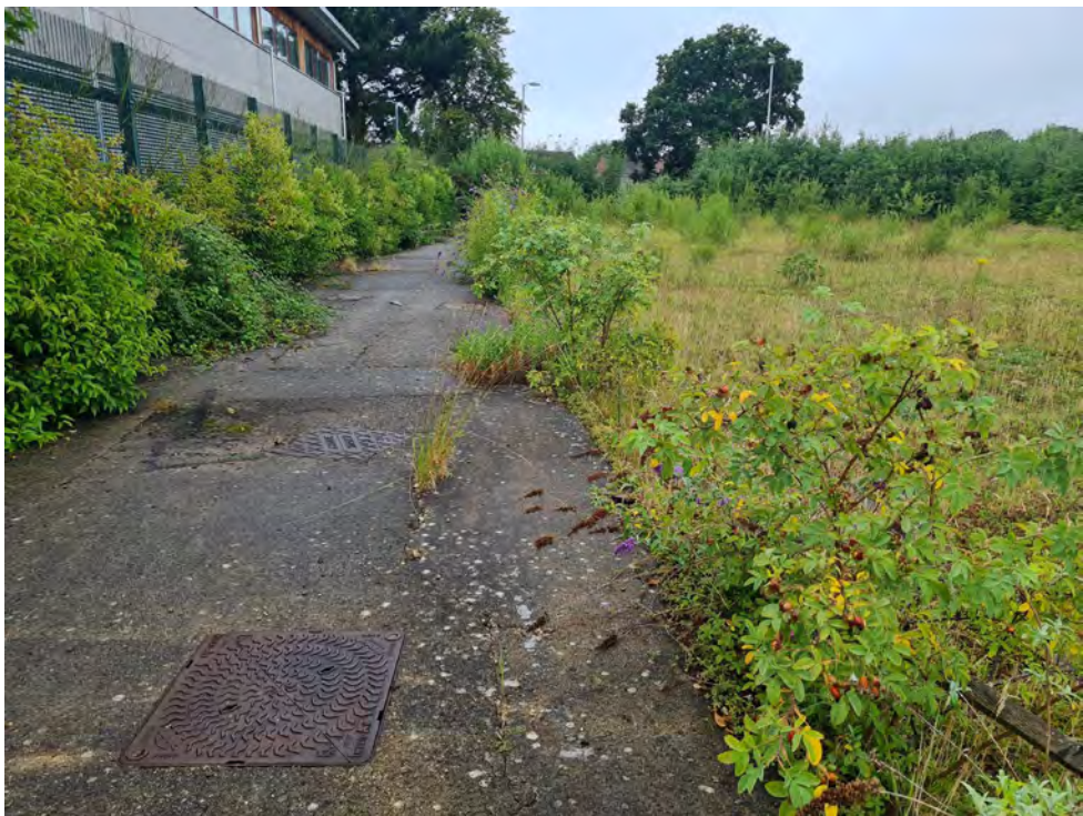
Plate 5: Many manhole covers and gulleys were located along the eastern edge of site. The south eastern corner was also overgrown with vegetation.
