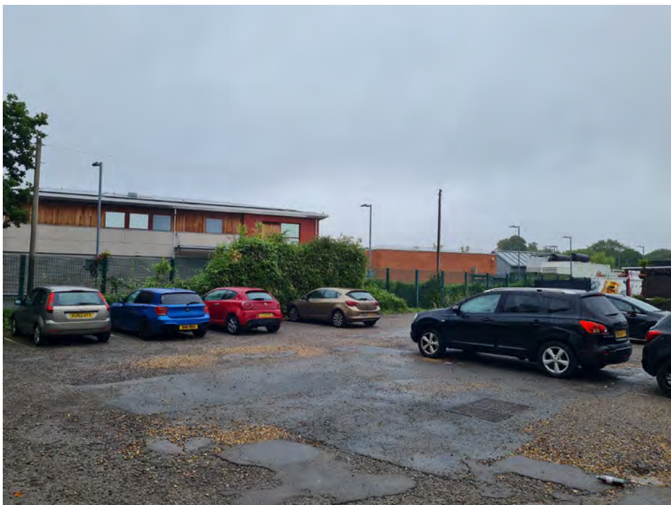
Plate 16: The SSE offices and electrical substation east of site are in the background of the image.
