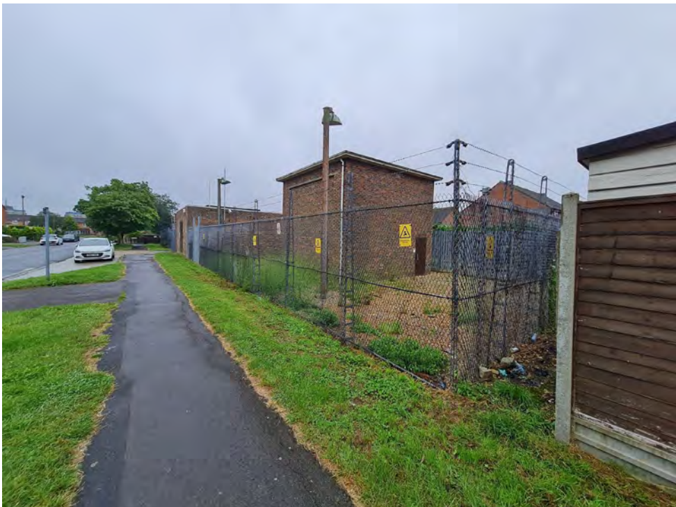
Plate 18: The electrical substation south of site.
