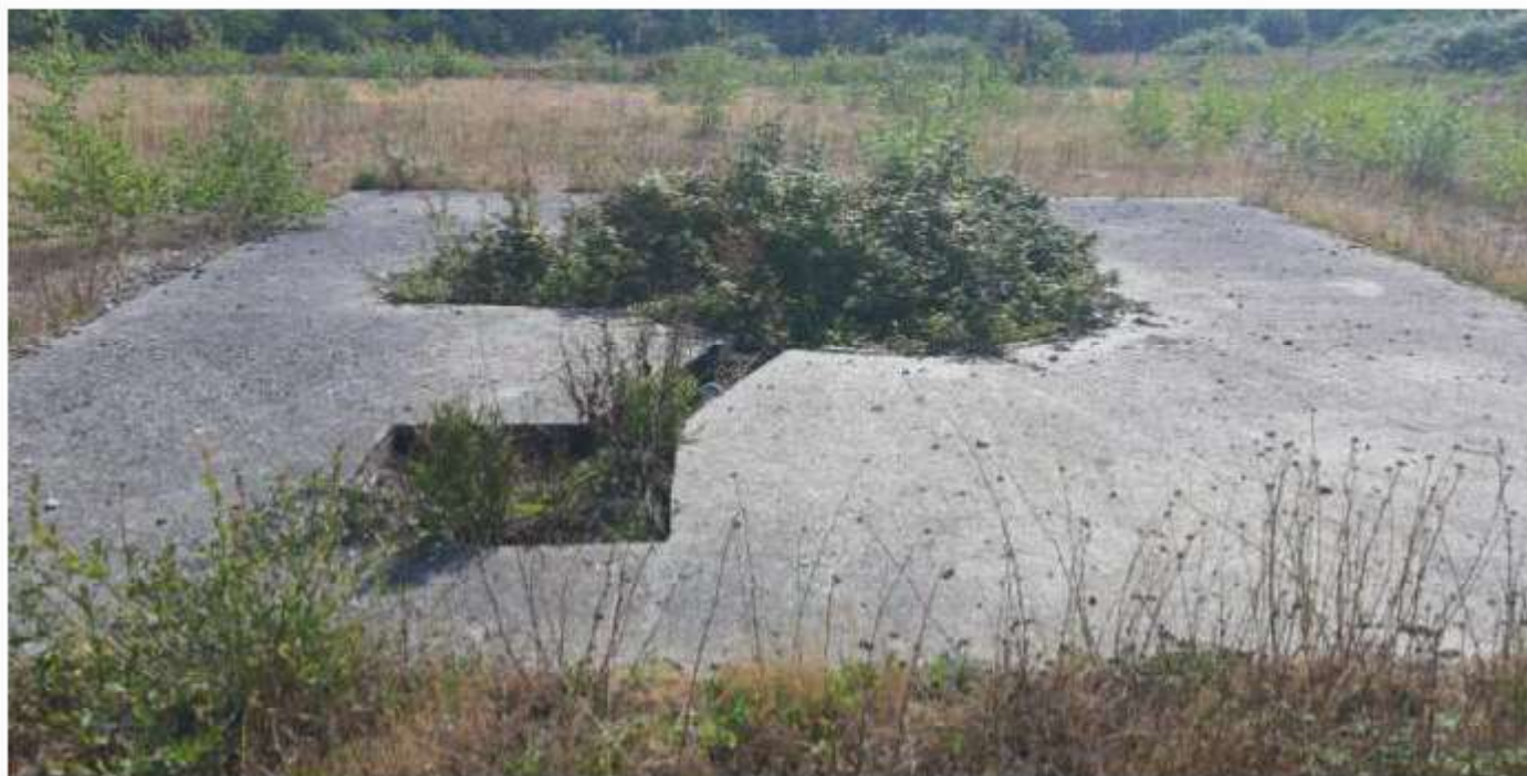
Plate 31 18b - Eastern concrete slab of the pair
