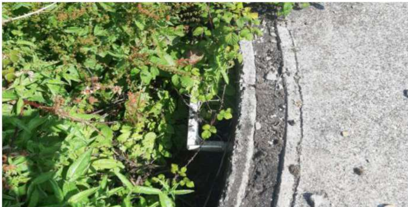
Plate 33 18d - Ladder rungs within the eastern slab hole (which was not completely infilled)
