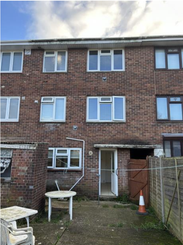
Rear view of 161 Park House Farm Way
