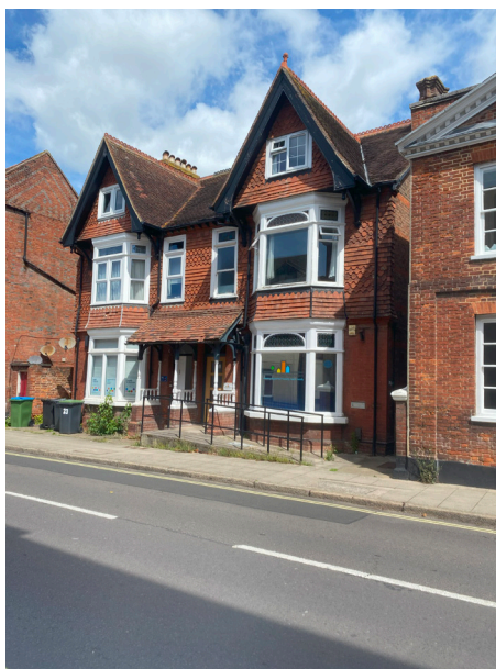
Image 06 Wide view of building, accommodating no.23/23A (left) and no.25/25A (right).
