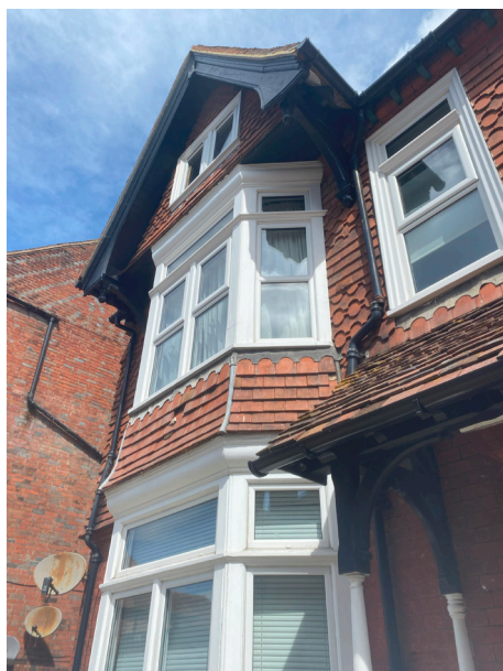
Image 05 Exterior view of UPVC windows of no.23 East Street.
