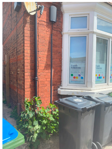
Image 07 UPVC bay windows on no.23 East Street.
