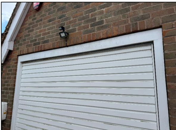
Photo 15: Garage door with no gaps
