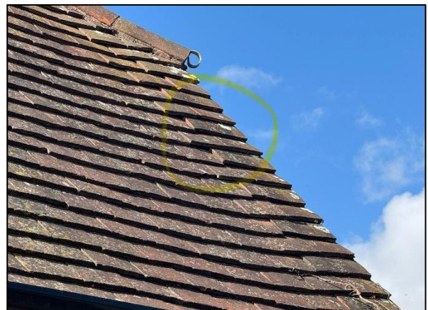
Photo 10: Lifted clay tiles on southeast corner
