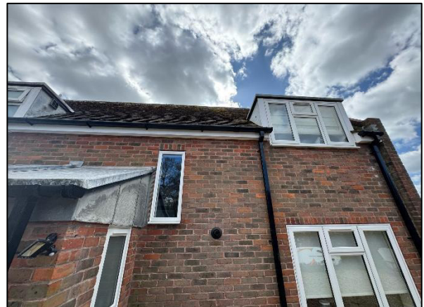
Photo 14: Sealed soffits on north elevation.
