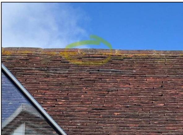
Photo 9: Lifted clay tiles near ridge on south elevation
