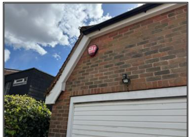
Photo 16: Sealed soffits at northeast corner
