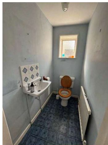
Figure 47: New window & fixtures.
