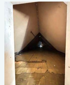
Figure 57: Storage within roof.
