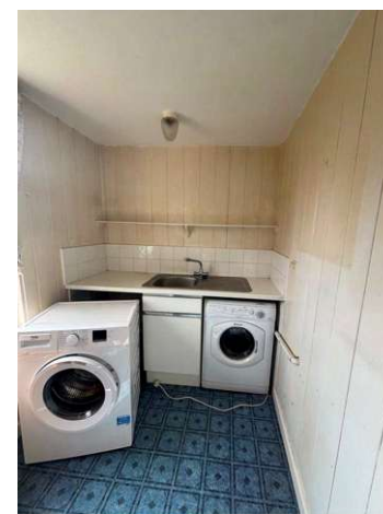
Figure 49: Appliances to be removed.
