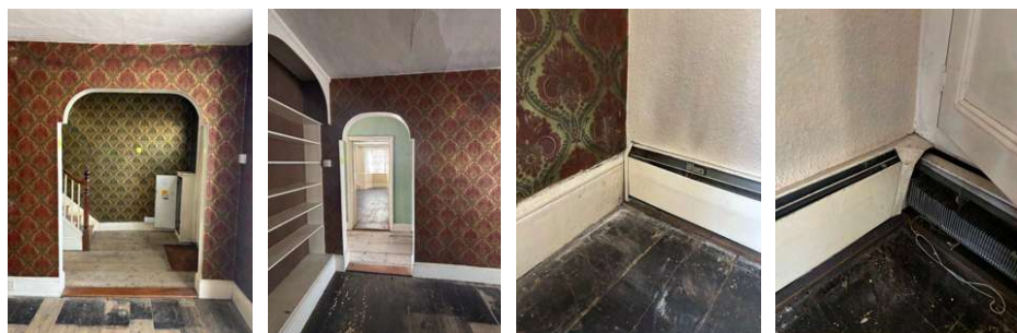
Figure 40 & 41: Archways to be turned into doors.
