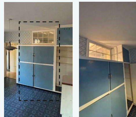
Figures 31 & 32: Existing Window between Kitchen & Larder.
