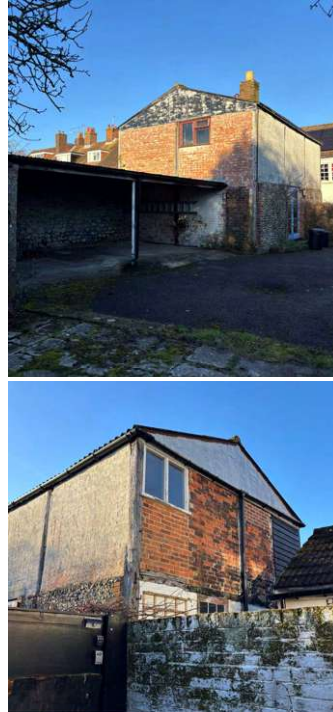
Figures 74 & 75: Existing Barn – External
