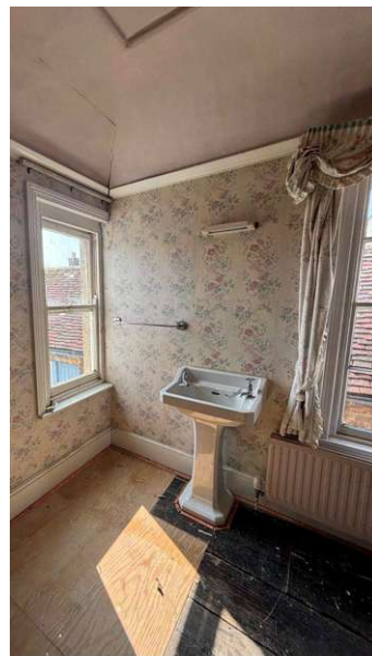
Figures 51: Existing Window & Sink to be removed.
