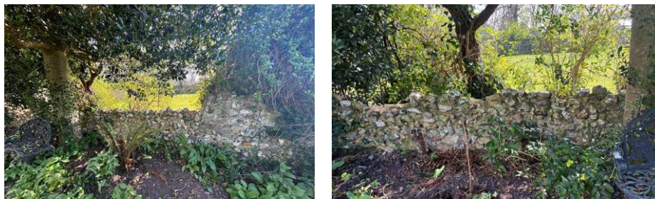
Figure 63 – 65: Existing rear garden wall.
