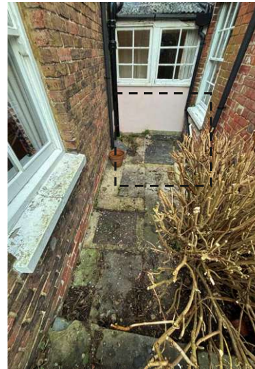
Figure 28: Coal Chute Area
