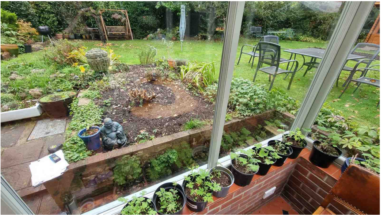
View from inside existing conservatory facing rear garden This shows the brickwork retaining wall that surrounds the existing conservatory
