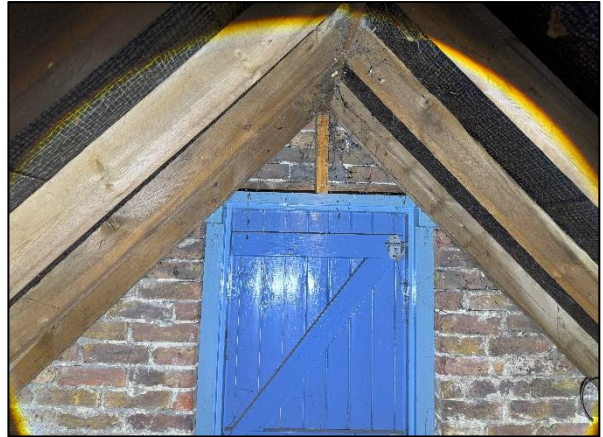
Photo 8: Interior loft void.
