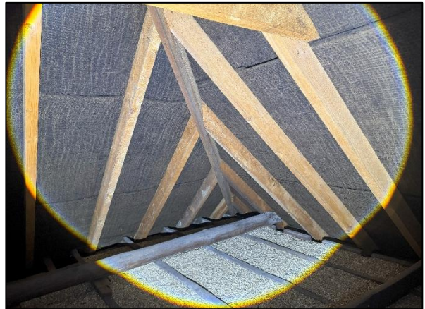
Photo 12: Interior loft void.
