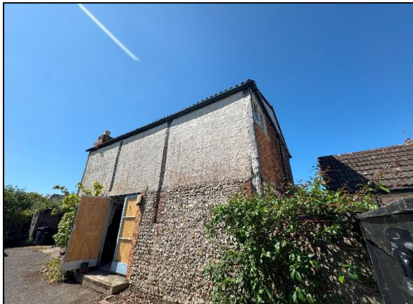
Photo 25: Barn east elevation.
