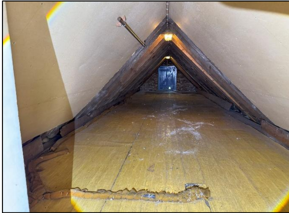
Photo 7: Interior loft void.
