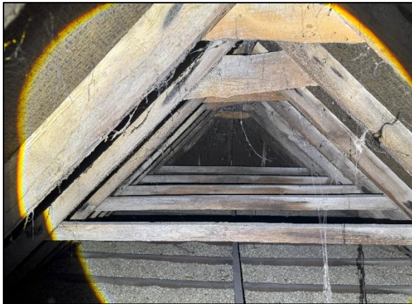
Photo 11: Interior loft void.
