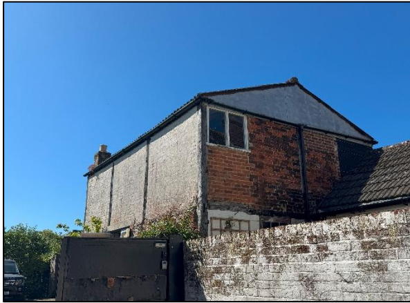
Photo 27: Barn north elevation.
