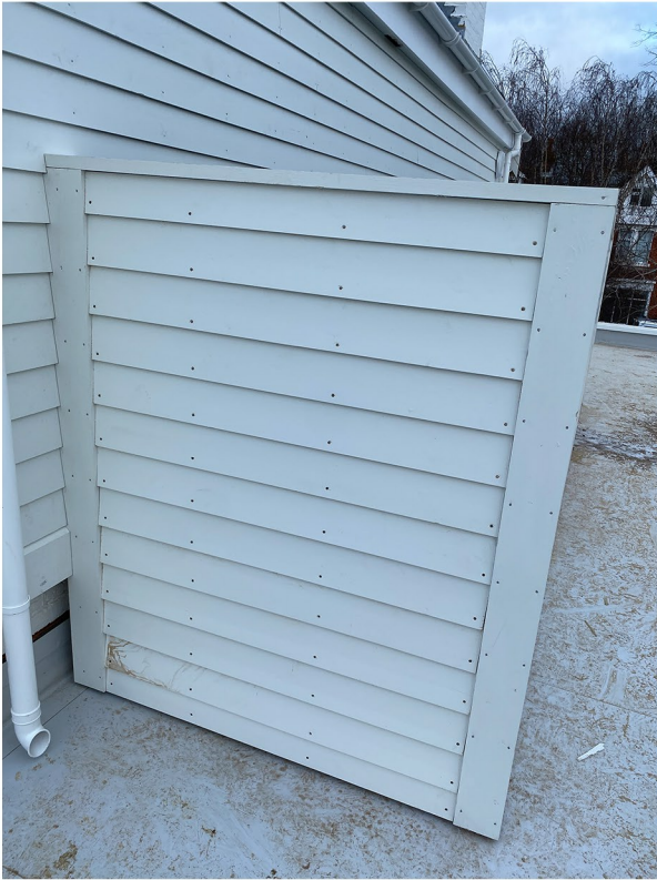
FIRST FLOOR VIEW - HOUSING FROM THE WEST
