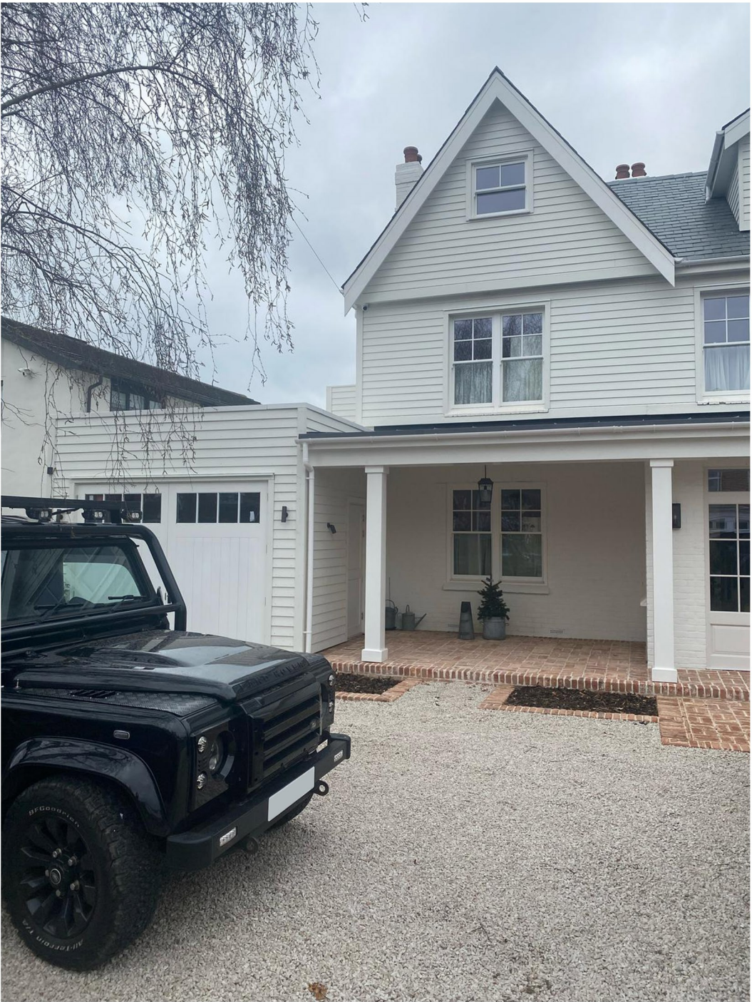
EAST VIEW FROM THE STREET
