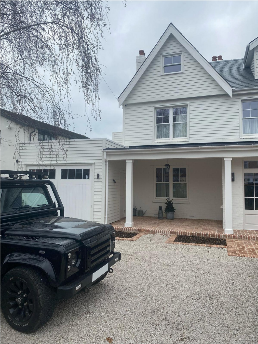
EAST VIEW FROM THE STREET
