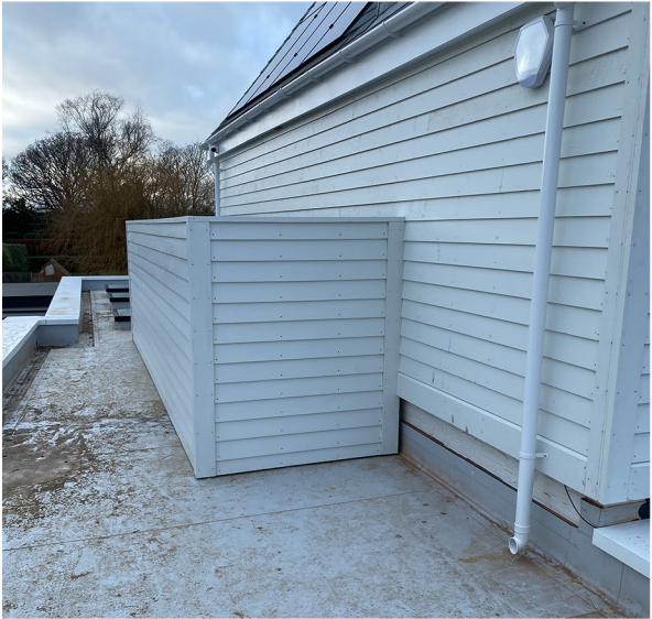
FIRST FLOOR VIEW - HOUSING FROM THE EAST
