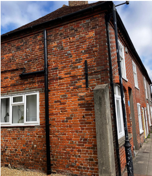
03 - Additional drainage pipe to the side facade. - Window replaced on the side facade
