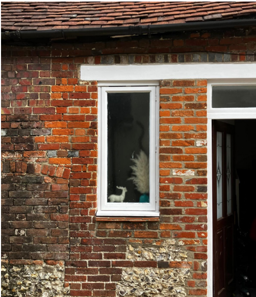
02 - Existing windows unchanged on side facade
