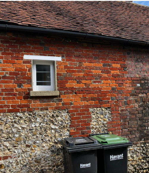
01 - Existing windows unchanged on side facade
